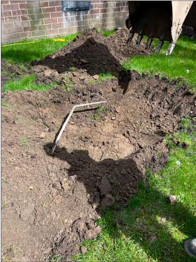
Looking north at an undocumented utility line at a shallow depth within the abandoned Trench 5.
