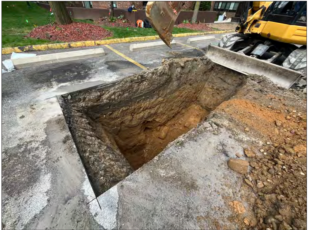
View of the western wall of Trench 2, where the disturbed fill layers were slightly shallower; note: the indentation in the wall is situated near the interface between the disturbed soils and the subsoil and was formed by the removal of a large cobble, seen in the trench to the right of the photograph.
