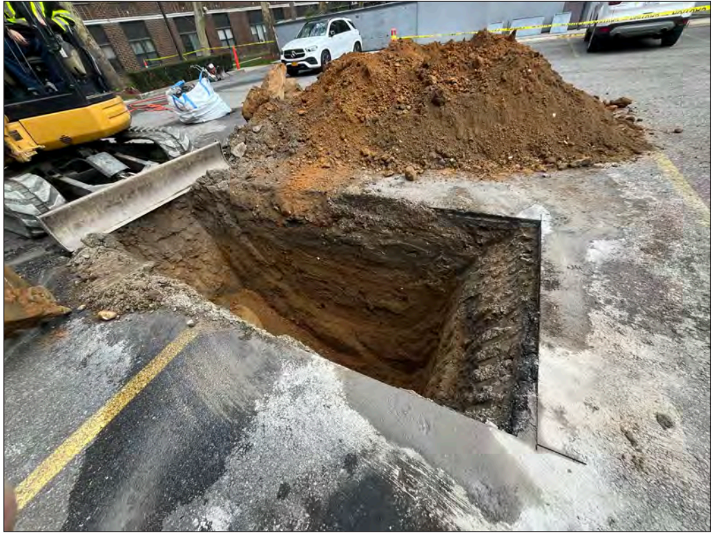
View of the eastern wall of Trench 2, showing the layers of disturbed fill between the pavement/bedding and the clean subsoil.
