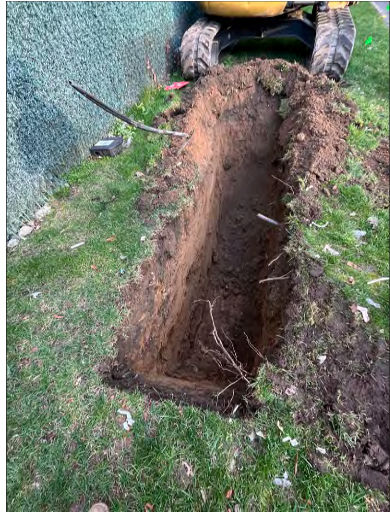
View north of Trench 1 after excavation, showing clean subsoil below the depth of the existing sod layer; a damaged sprinkler line is visible on the left side of the photograph.
