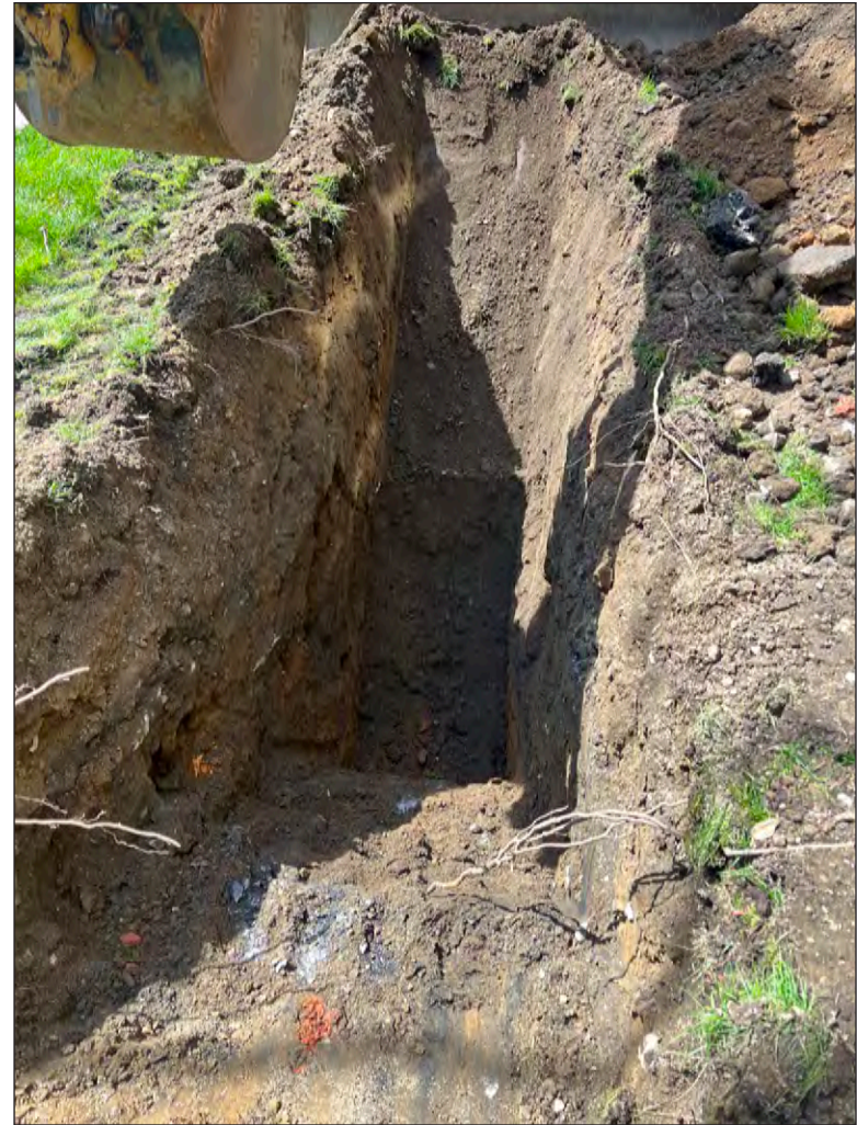
Looking west at Trench 4, showing densely packed disturbed soils throughout the entire depth of the trench; project-related impacts in this area will not exceed the depth of disturbed soils.
