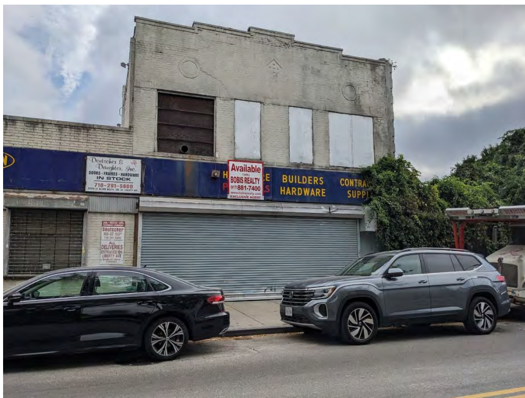
Photograph 25. Block 10112, Lot 68 showing a two-story building. View looking northeast from 150 th Street.
