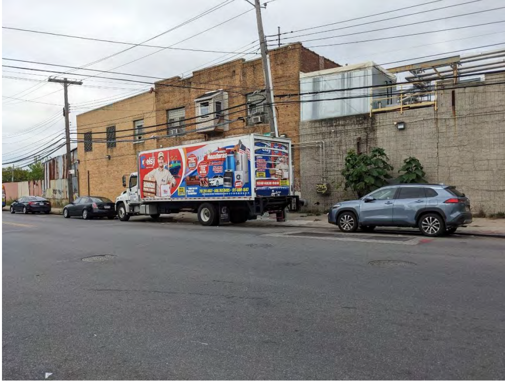
Photograph 31. Block 10115, Lot 53, showing two buildings from the former Elmhurst Dairy facility complex. View looking northwest from Tuskegee Airmen Way.
