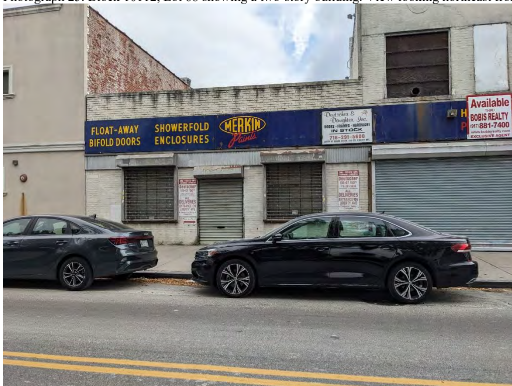
Photograph 26. Block 10112, Lot 70 showing a one-story building. Lot 18, which also has a one-story building, is located to the northeast of Lot 70 but does not front on a publicly accessible street. View looking northeast from 150 th Street.
