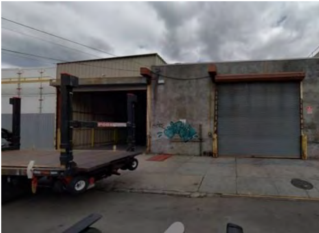
Photograph 18. Block 10107, Lot 73, showing one-story structure with garage door on left. View looking northeast from 150 th Street.
