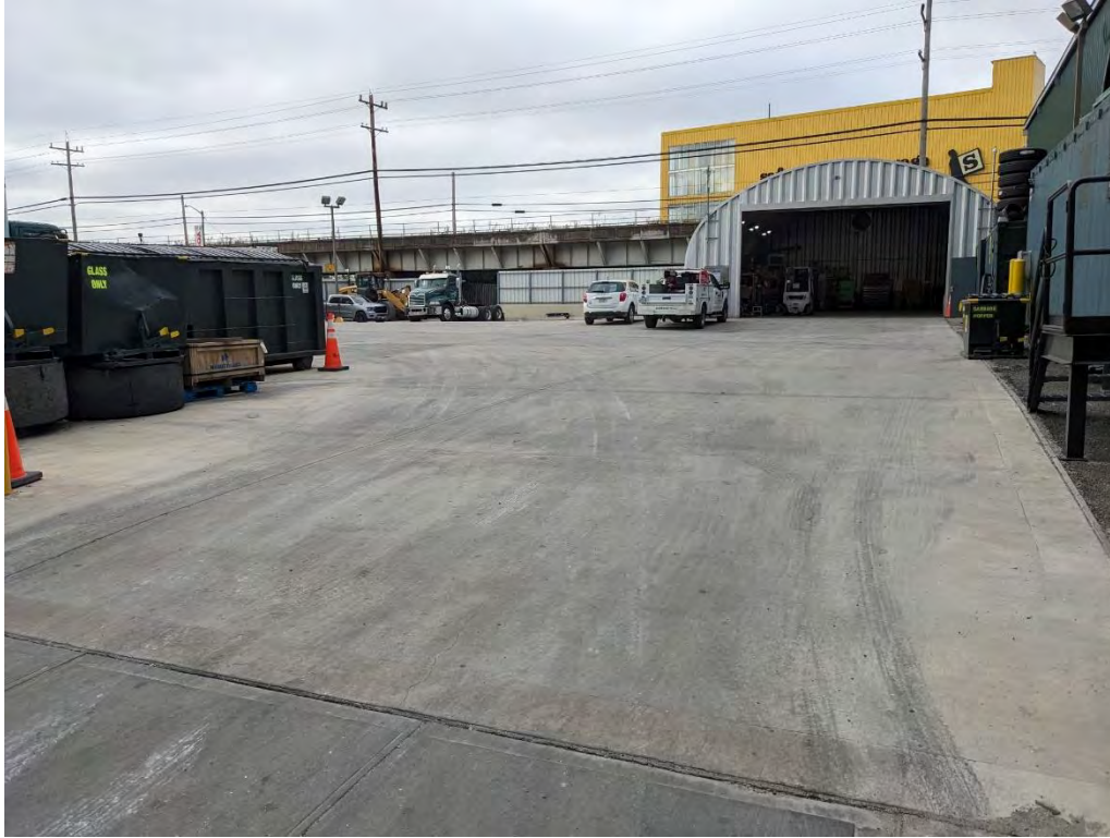
Photograph 21. Block 10109, Lot 31 showing the paved lot. View looking southwest from 158 th Street.
