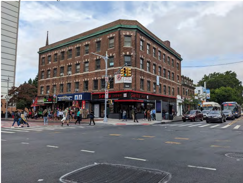
Photograph 14. Block 9754, Lot 34 showing the four-story with basement building in the center and the three-story with basement building on the right. View looking northwest from Jamaica Avenue and Parsons Boulevard.
