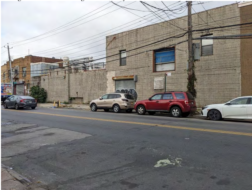
Photograph 30. Block 10115, Lot 53, showing two buildings from the former Elmhurst Dairy facility complex. View looking northwest from Tuskegee Airmen Way.
