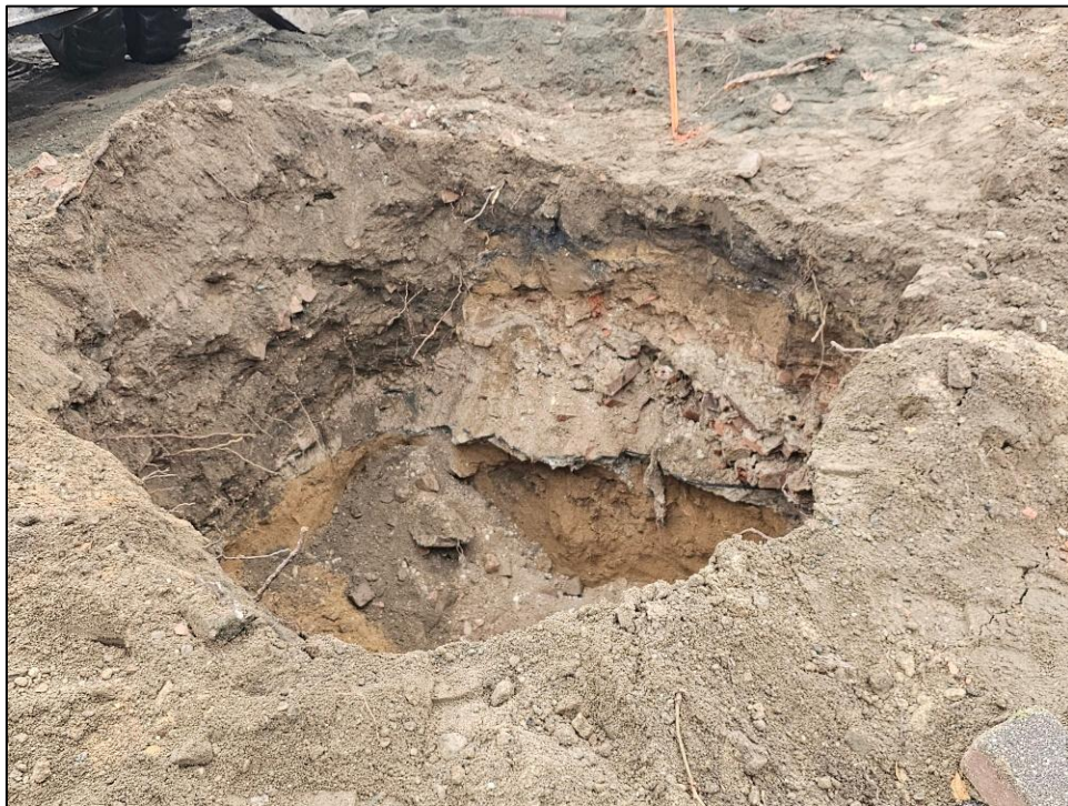
Image 6: Clean sand fill beneath the concrete floor in CB5.
