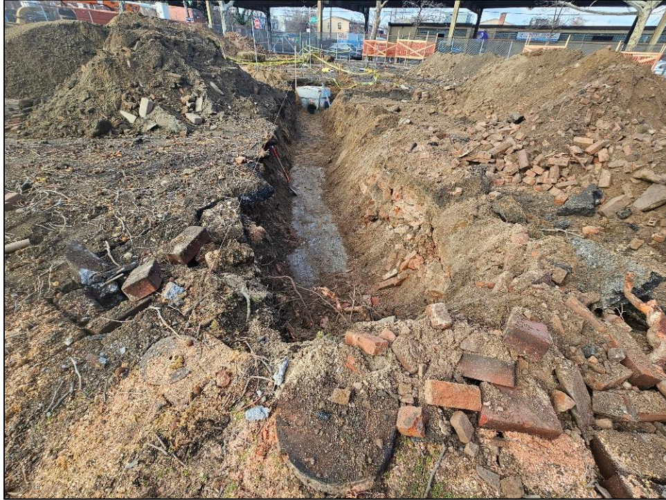
Image 13: Fully exposed concrete floor, connection trench from existing CB to CB4.
