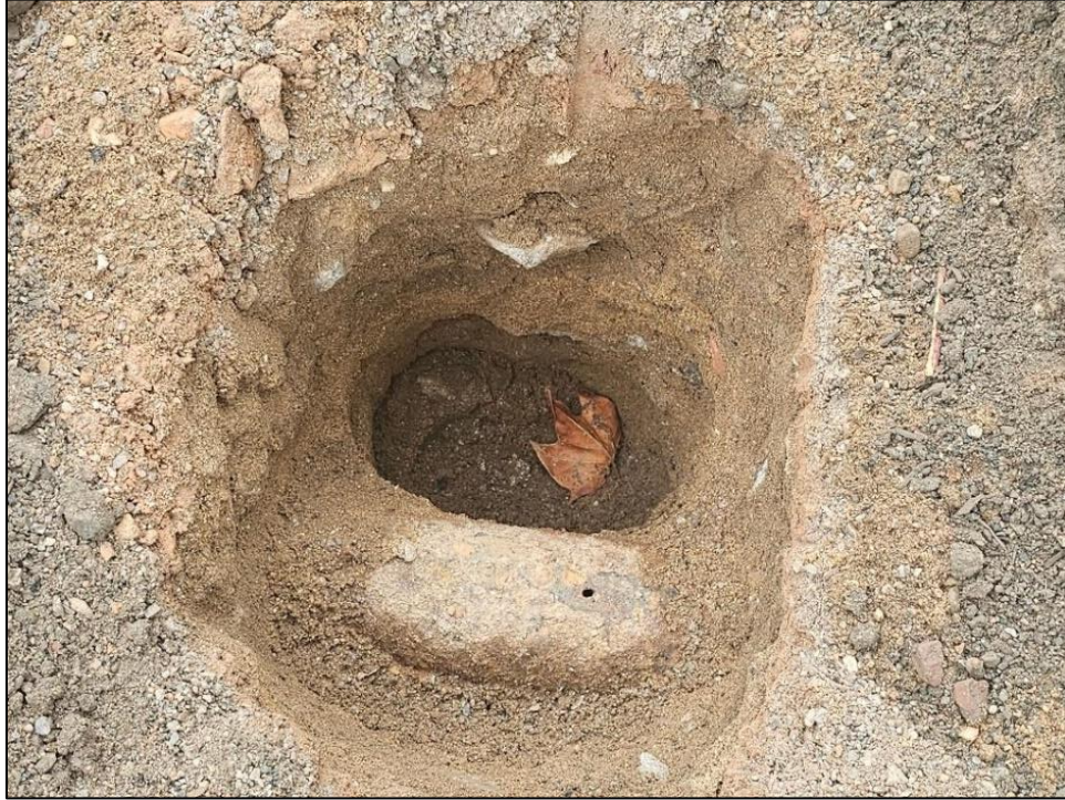
Image 29: Example of fill soils in pier pit 5.
