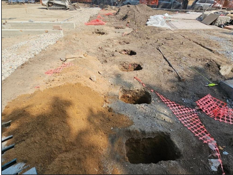
Image 31: Excavation for pier pits, looking north.
