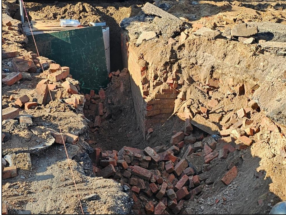
Image 19: Section of brick wall left in situ in trench connecting existing CB and CB3.
