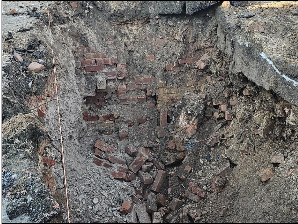
Image 17: In situ brick wall running north-south, located 10' from existing CB.
