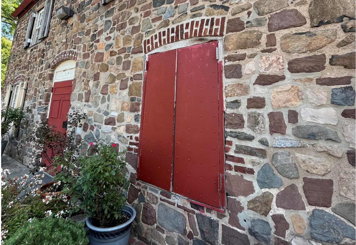
Photo 4. Metal-clad shutters on the ground floor of the original south (now west) façade. View northeast.
