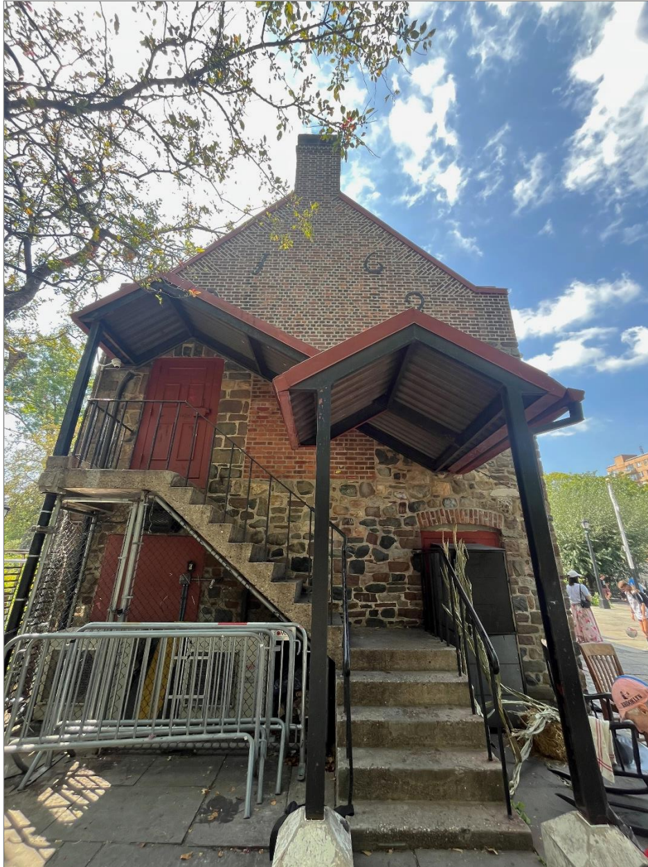
Photo 5. Present-day north façade, which was originally the west façade. The 1930s pavilion was attached to this façade. The fire escape is a later addition. This façade will be impacted by the upcoming addition and renovations and will be the site of the new accessible entrance. View south.
