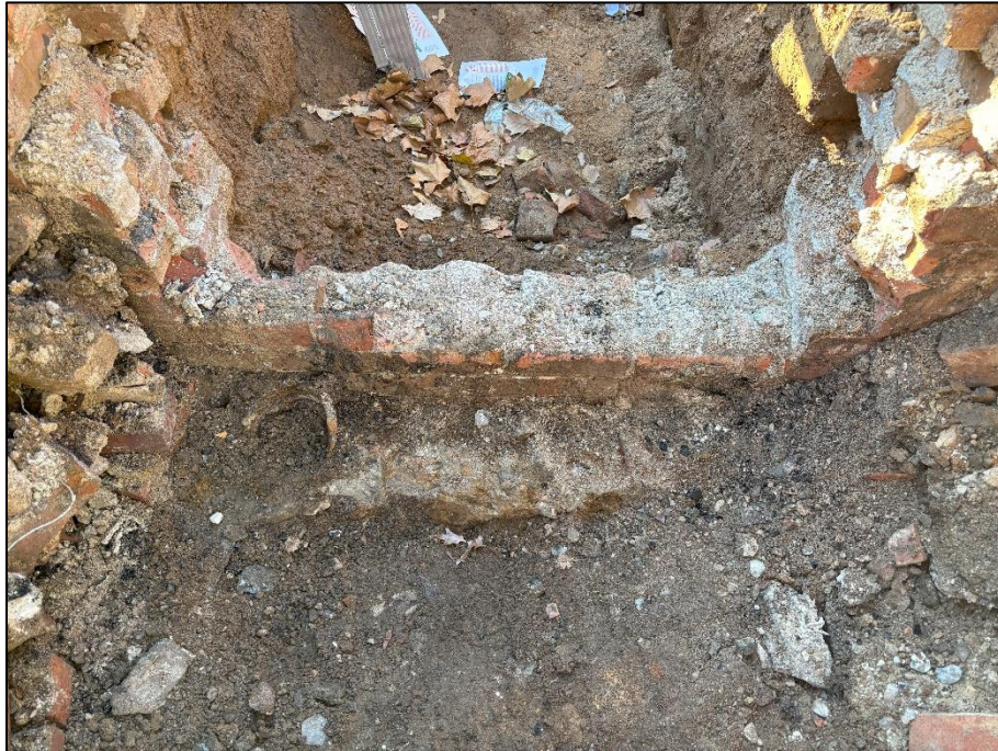
Plate 5: Close up of brick footing and pipe.
