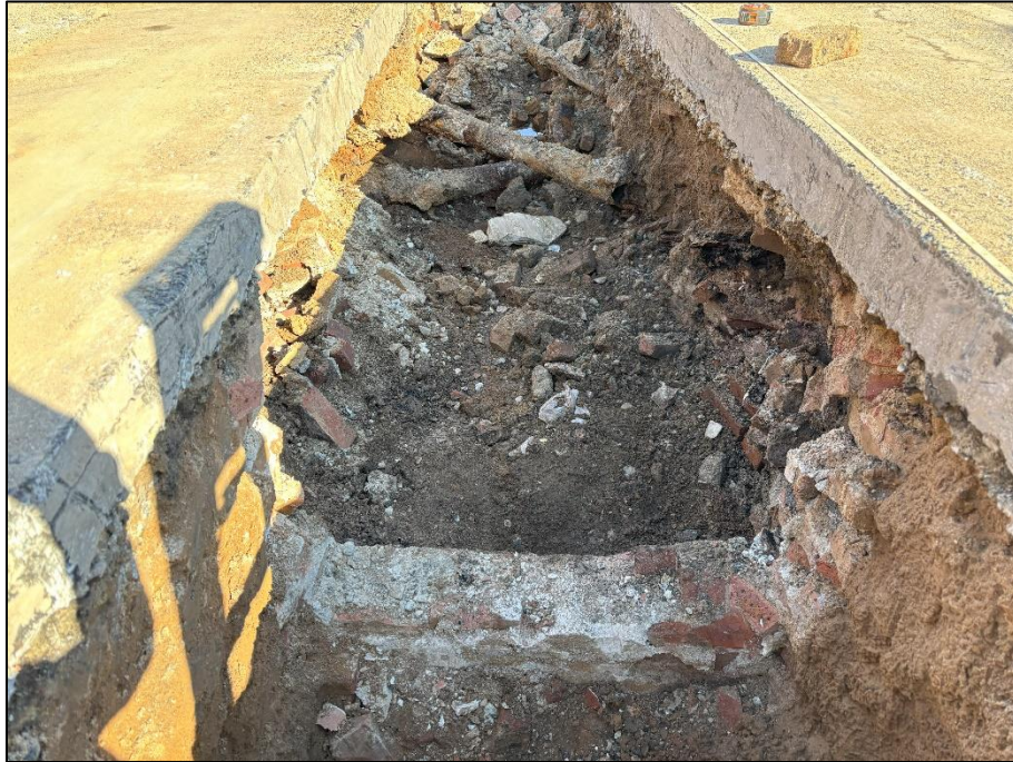
Plate 3: Brick footing with pipes in background.
