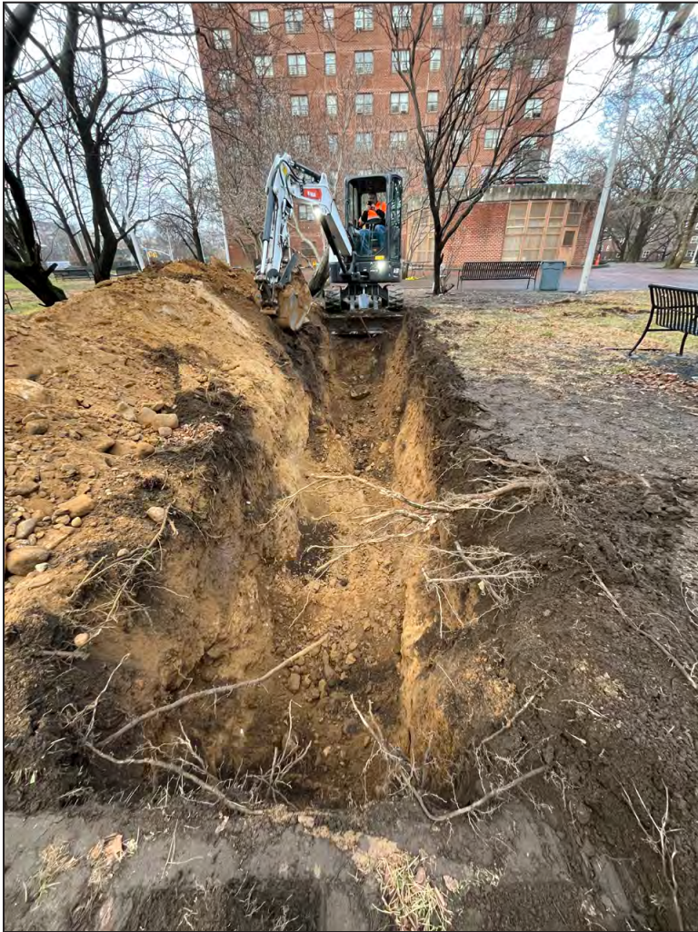
Looking west at completed Trenches 2 (foreground) and 3 (background), showing a consistent soil profile across the excavation
