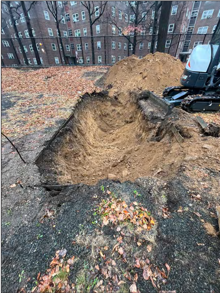
Looking east at Trench 1 following excavation; showing iron plates/ planter boxes within topsoil and underlying layers of subsoil 1
