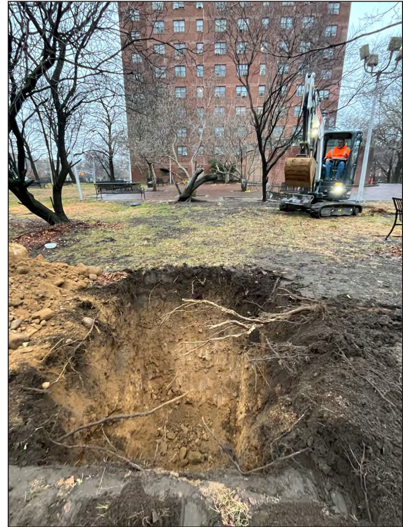
Looking west at excavated Trench 2; Trench 3 was opened in a continuous line to the west 2
