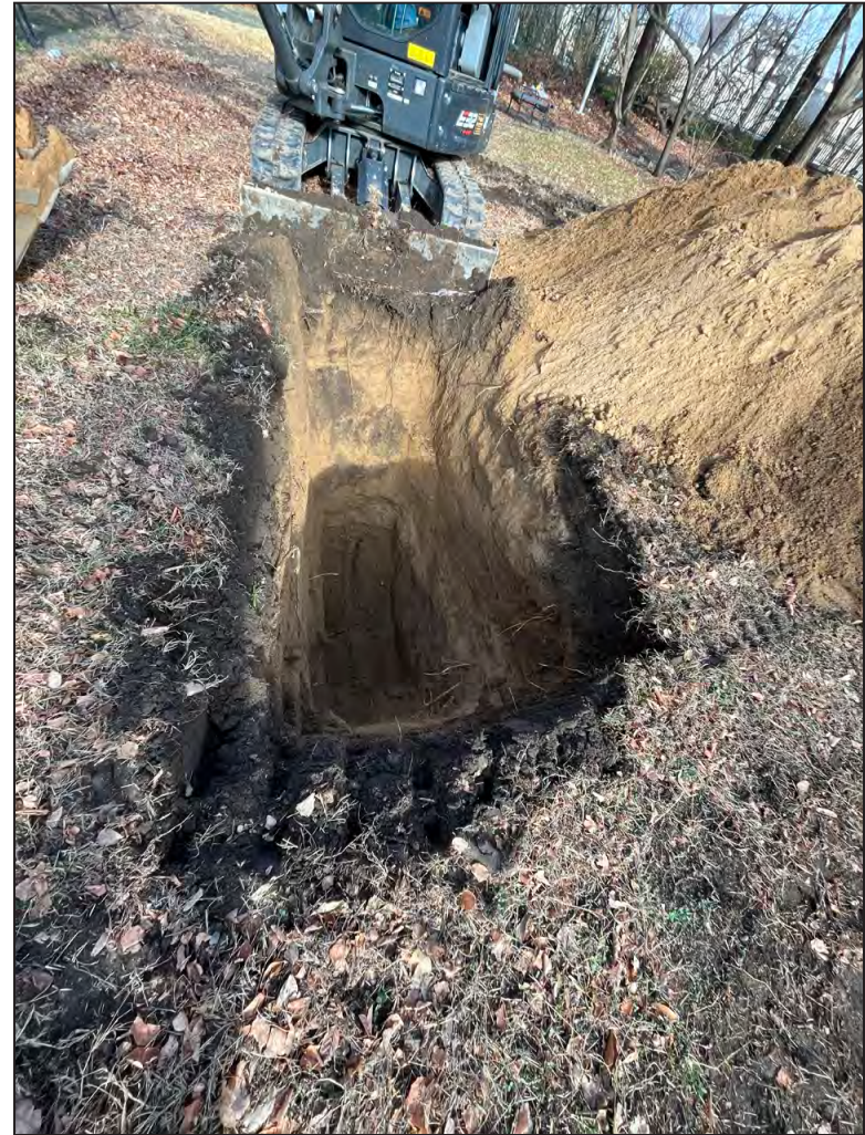
Looking north at Trench 4, which contained clean sandy fill to a depth of at least 9 feet
