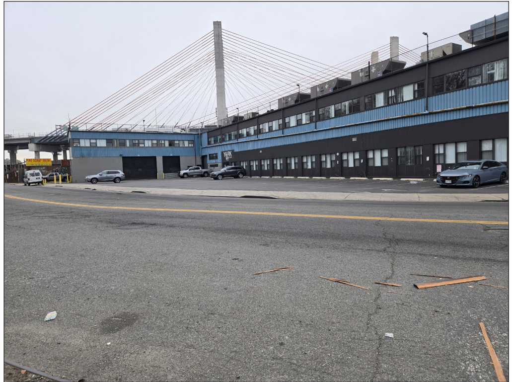
Looking northeast along Laurel Hill Boulevard, with Block 2560, Lot 6 in the foreground and the vacant lot on Lot 22 in the distance
