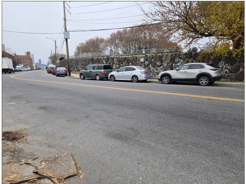
Looking northwest at the retaining wall lining the southern side of Calvary Cemetery along Review Avenue, showing grave markers at a higher elevation
