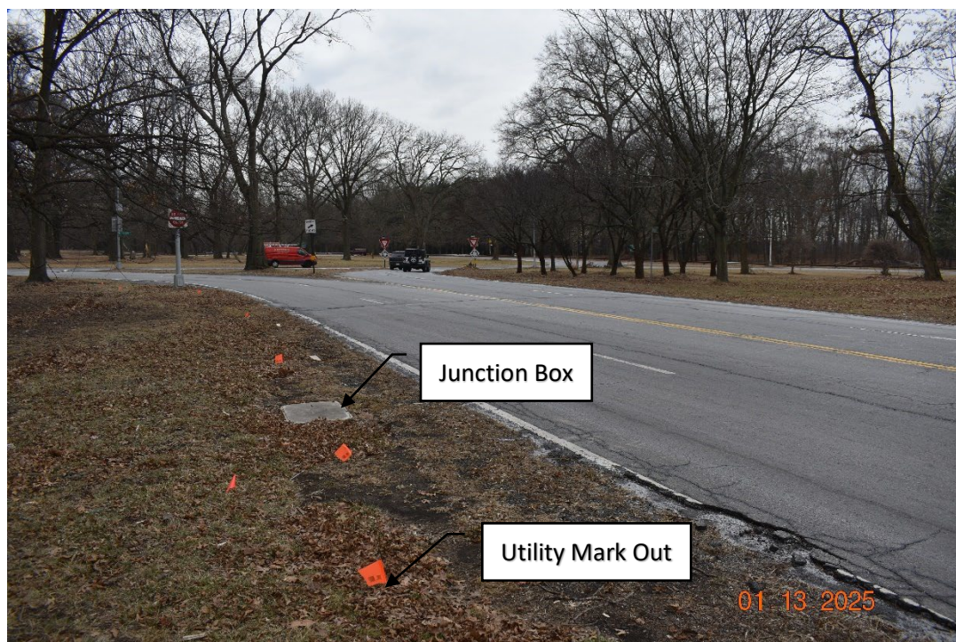
Photograph 30. View of the STs 68 and 69 with utility mark out. Facing southwest (NC 1/13/2025).
