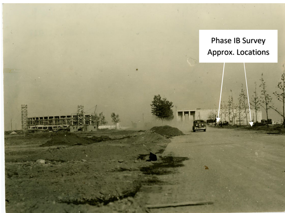
Figure 6. Photograph with a date range of 1934-1945 shows the construction of Orchard Beach Bath House and Promenade. The Phase IB Survey location can be seen in this photograph near the rows of trees (NYC Municipal Archives 1934-1945).
