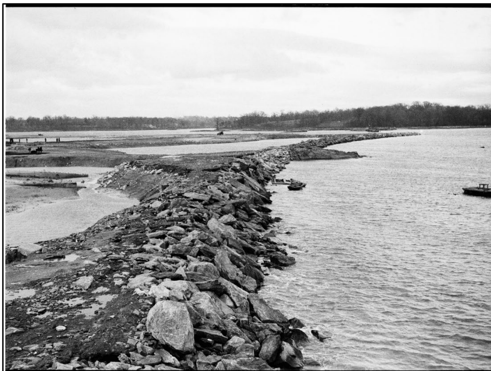
Figure 5. View of the construction of Orchard Beach seawall in 1935 (NYC Municipal Archives 1935).
