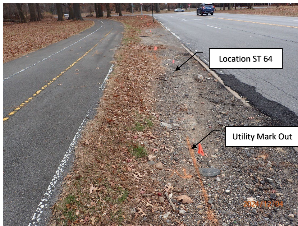
Photograph 29. View of ST 64 in line with communication utility located at the southern end of the Phase IB Survey. Facing south. (LC 12/4/2024)
