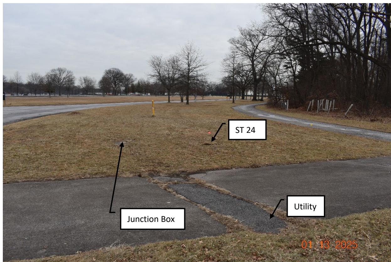
Photograph 13. View of ST 24 and evidence of a buried utility. Facing north. (NC 1/13/2025).
