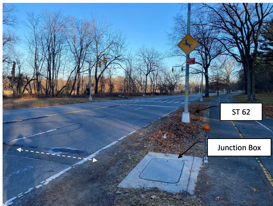
Photograph 28. View of utility (white dashed line) and junction box located between STs 62 and 63. ST 63 is not visible in the photograph. Facing north (NC 12/4/2024)
