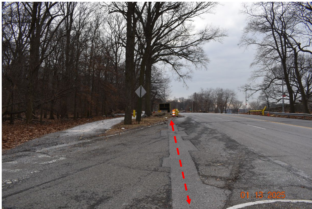
Photograph 17. Indication of a buried utility (red dashed line). Facing south (NC 1/13/2025).
