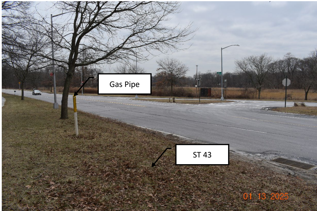
Photograph 22. View of a gas pole near the location of ST 43. Facing southwest (NC 1/13/2025).
