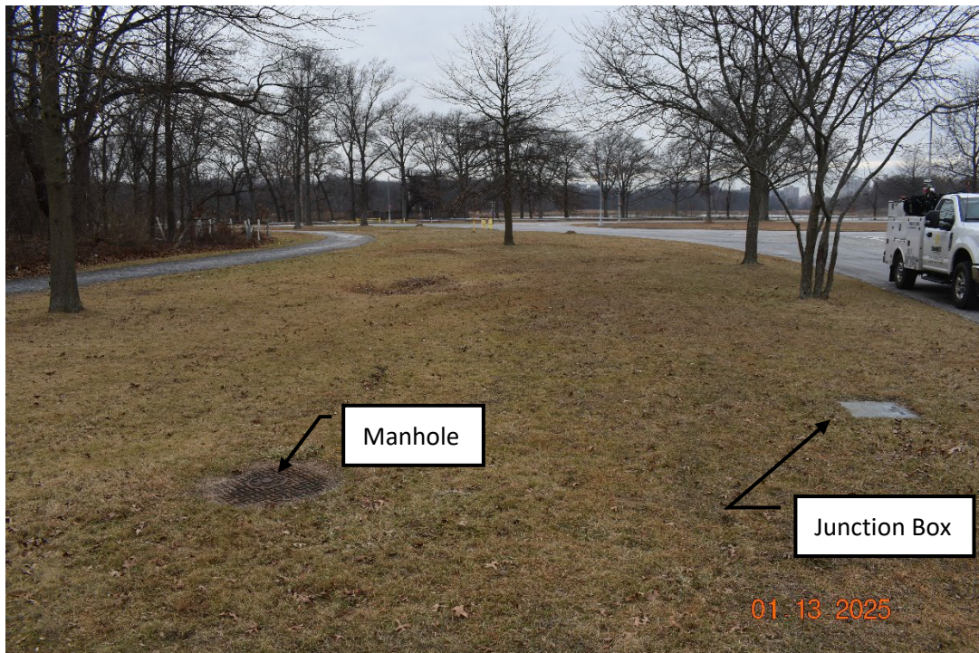
Photograph 12. View of manhole and junction box near ST 20 location. Facing east. (NC 1/13/2025)
