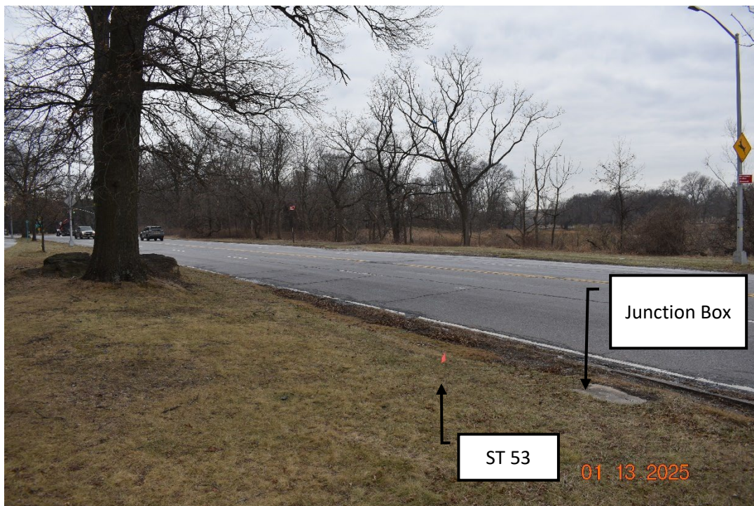
Photograph 26. Location of ST 53 near junction box. Facing southwest (NC 1/13/2025).
