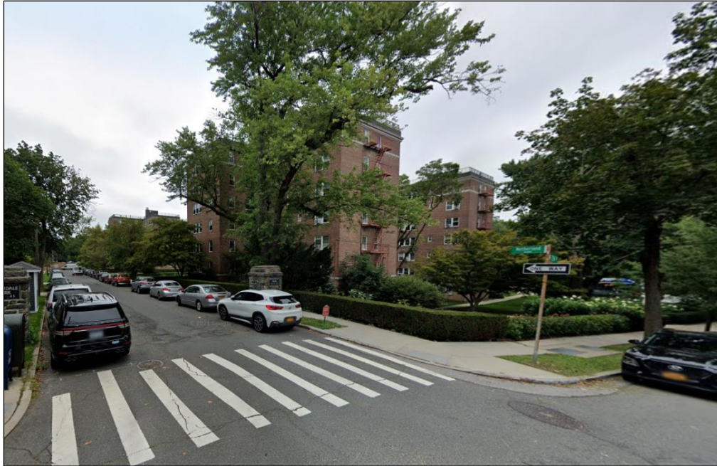
Figure 5-View of Riverdale Park Apartments showing south elevation of sections A and B, looking northeast showing tree cover.
