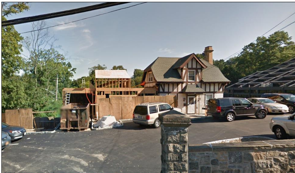
Figure 8: View of Gatehouse in 2011 With New Additions Under Construction, Facing North (GoogleMaps 2024).
