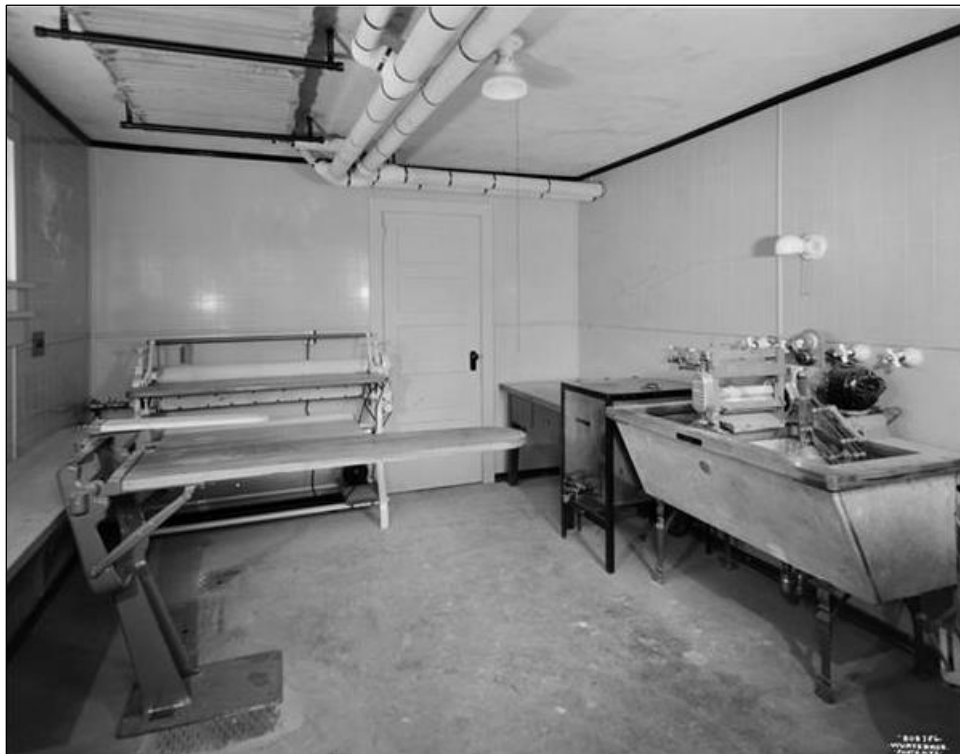
Figure 30- View of onsite laundry room circa 1942 (Wurts Brothers 1942).
