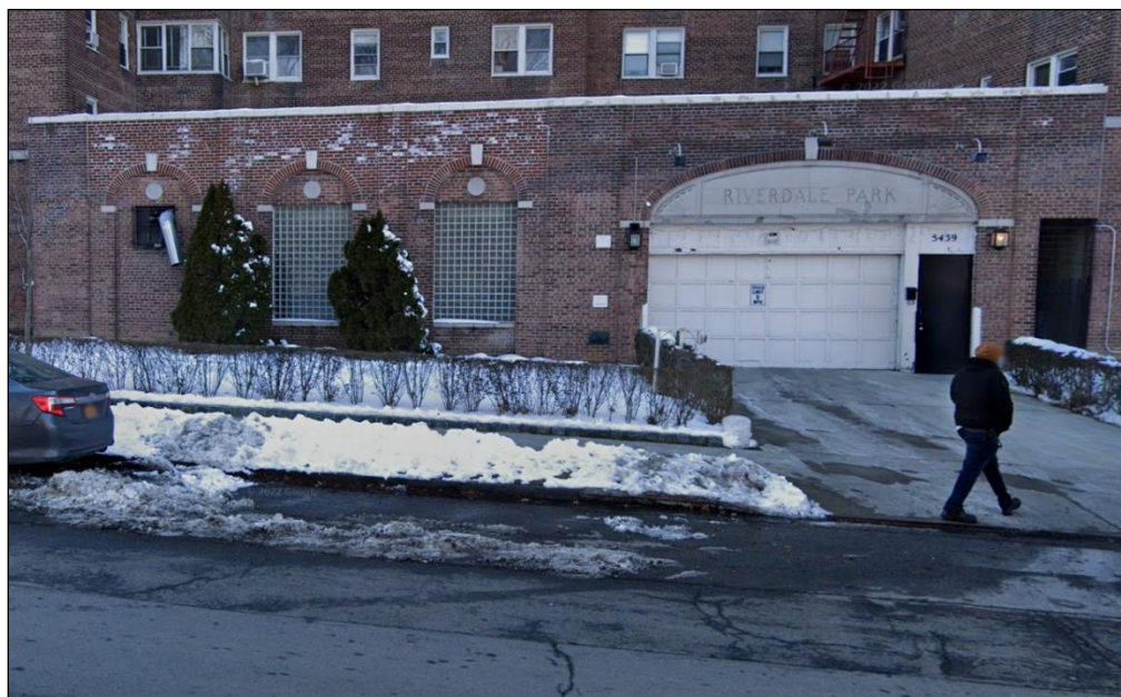
Figure 12-Detail view of original garage entrance that retains the wooden garage door, and entry button. The segmental brick arches with cast stone keystones are one of the remaining colonial revival elements on
