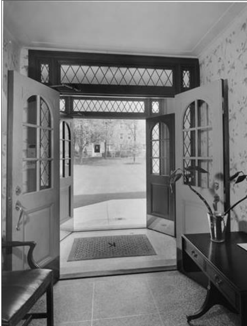
Figure 15- View of entry foyer into Building K showing original doors, windows, floor, and wallpaper circa 1942 (Wurts Brothers 1942).
