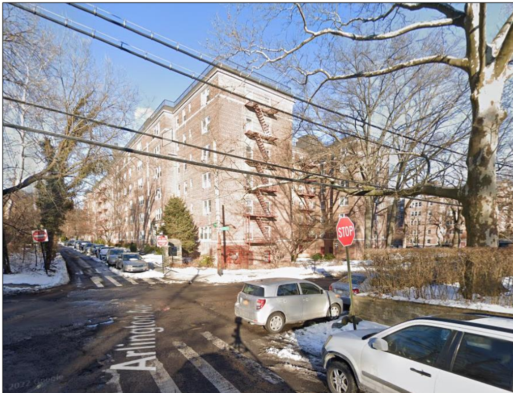
Figure 6- View of Riverdale Park Apartments showing south elevation of sections J and K, looking northeast showing tree cover.
