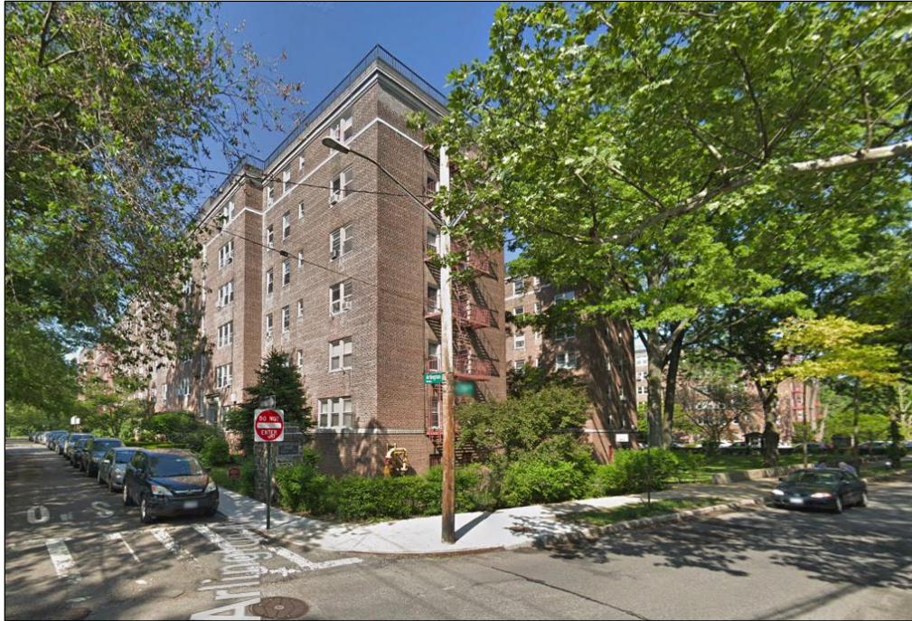
Figure 7-View of Riverdale Park Apartments showing south elevation of sections J and K, looking northeast showing tree cover.
