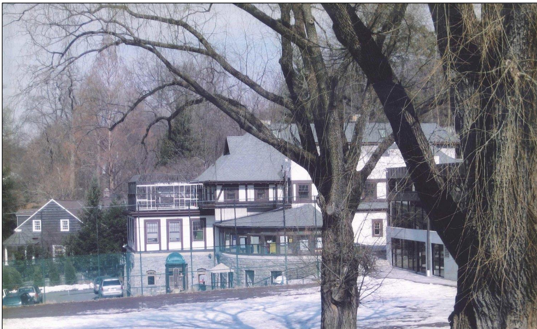
Figure 12: View of Historic Carriage House (Eidman 2019).
