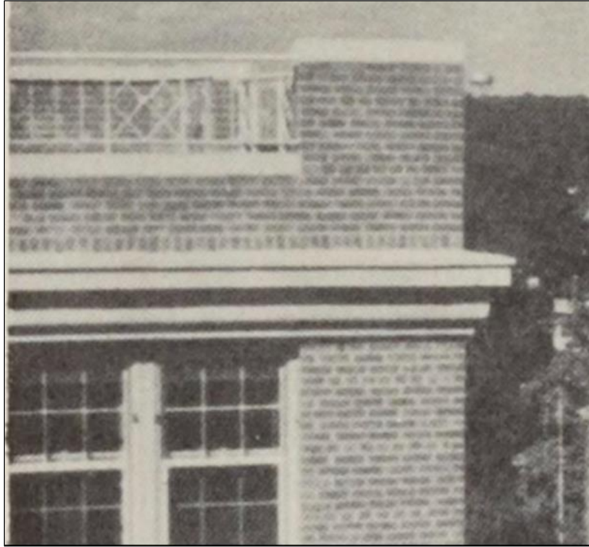
Figure 11- Detail showing original crenelation at the roofline with decorative railings (Riverdale Park, Inc 1940).
