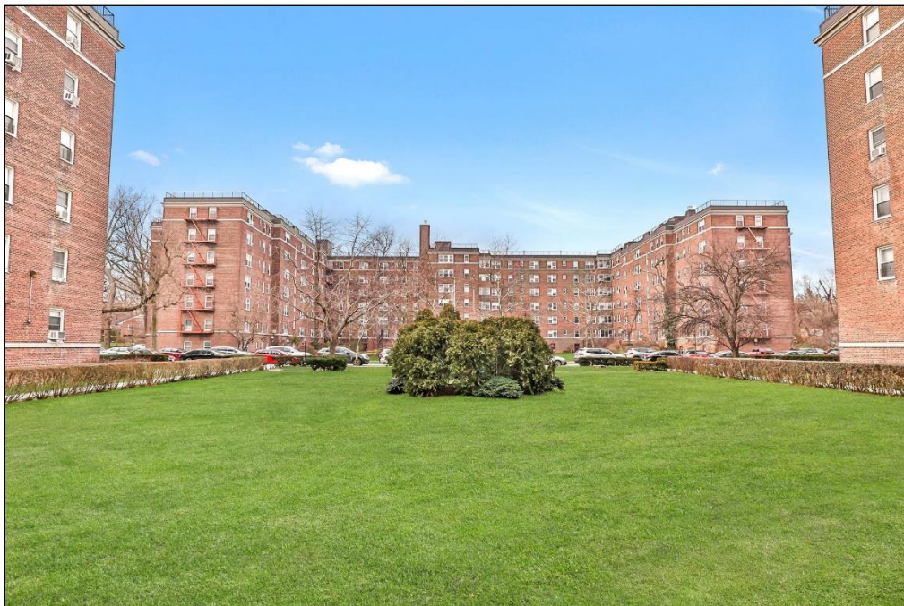
Figure 8- View of Riverdale Park Apartments showing east elevation of sections F,G,H,J, and K, looking east (Treabach Reality 2020)
