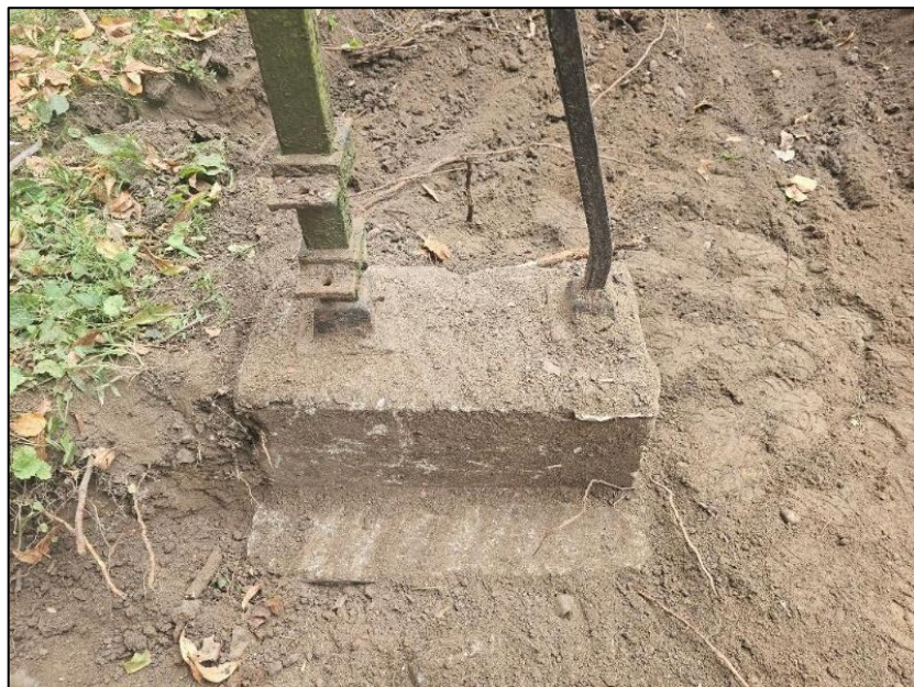
Image 1: Example of fence post footing.
