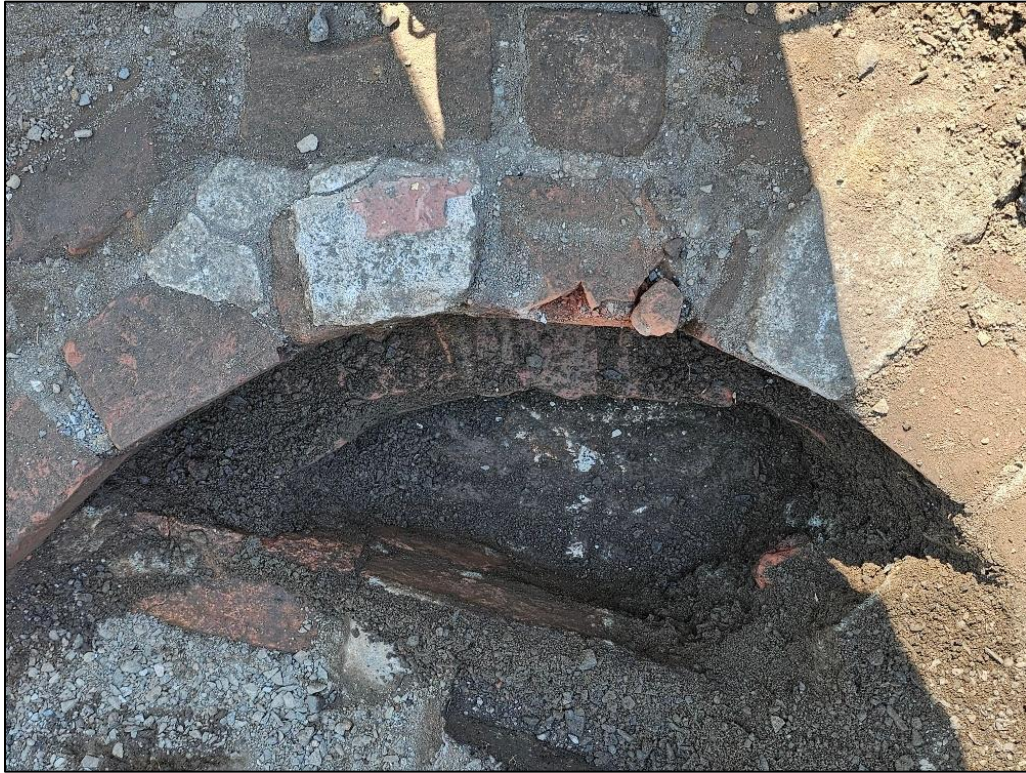
Image 3: Feature interior showing cement base at 20".
