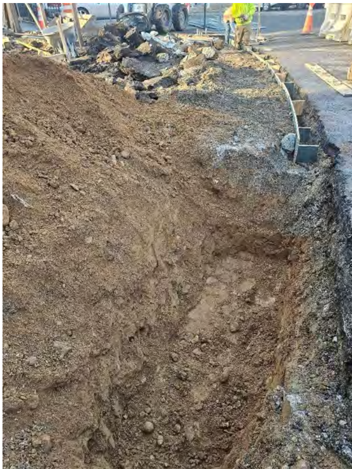
Photograph 12. Area 2, Excavated Tree Pit and full curb cut in background, view looking north.
