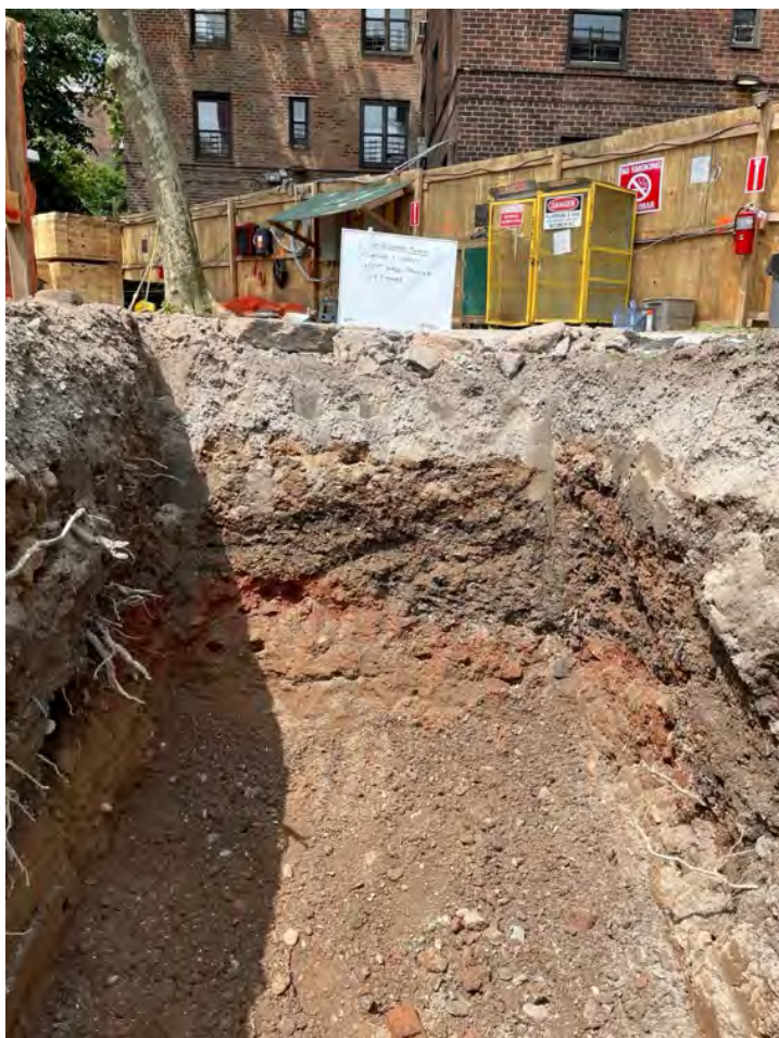
Photograph 15. Area 3, West Wall of the Support of Excavation Trench, showing limited remnants of the truncated brick feature at the southeast corner and north wall.
