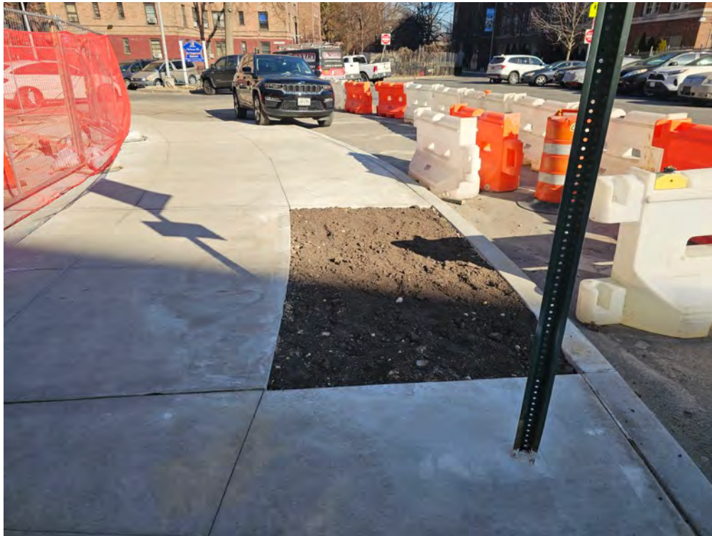
Photograph 13. Area 2, Filled Tree Pit and repaved sidewalk and curb, view looking north.
