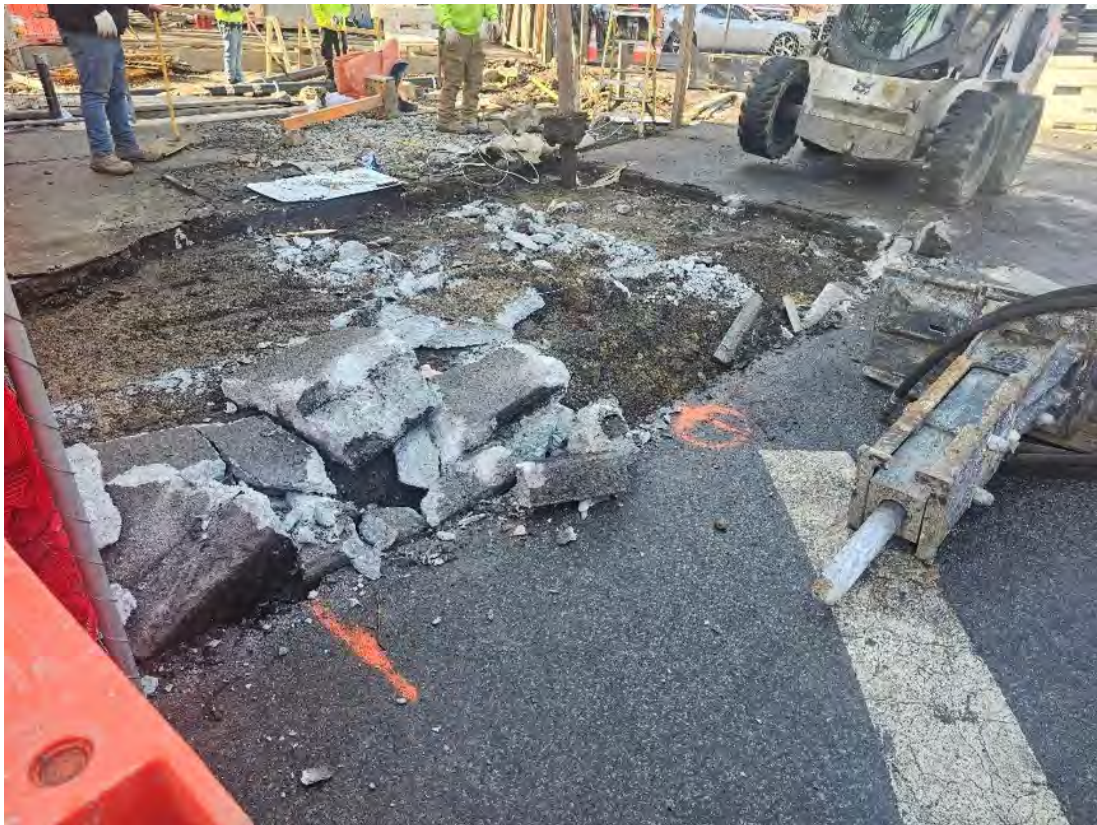
Photograph 9. Area 2, Tree Pit during the removal of the concrete sidewalk, exposing a thick fill stratum.
