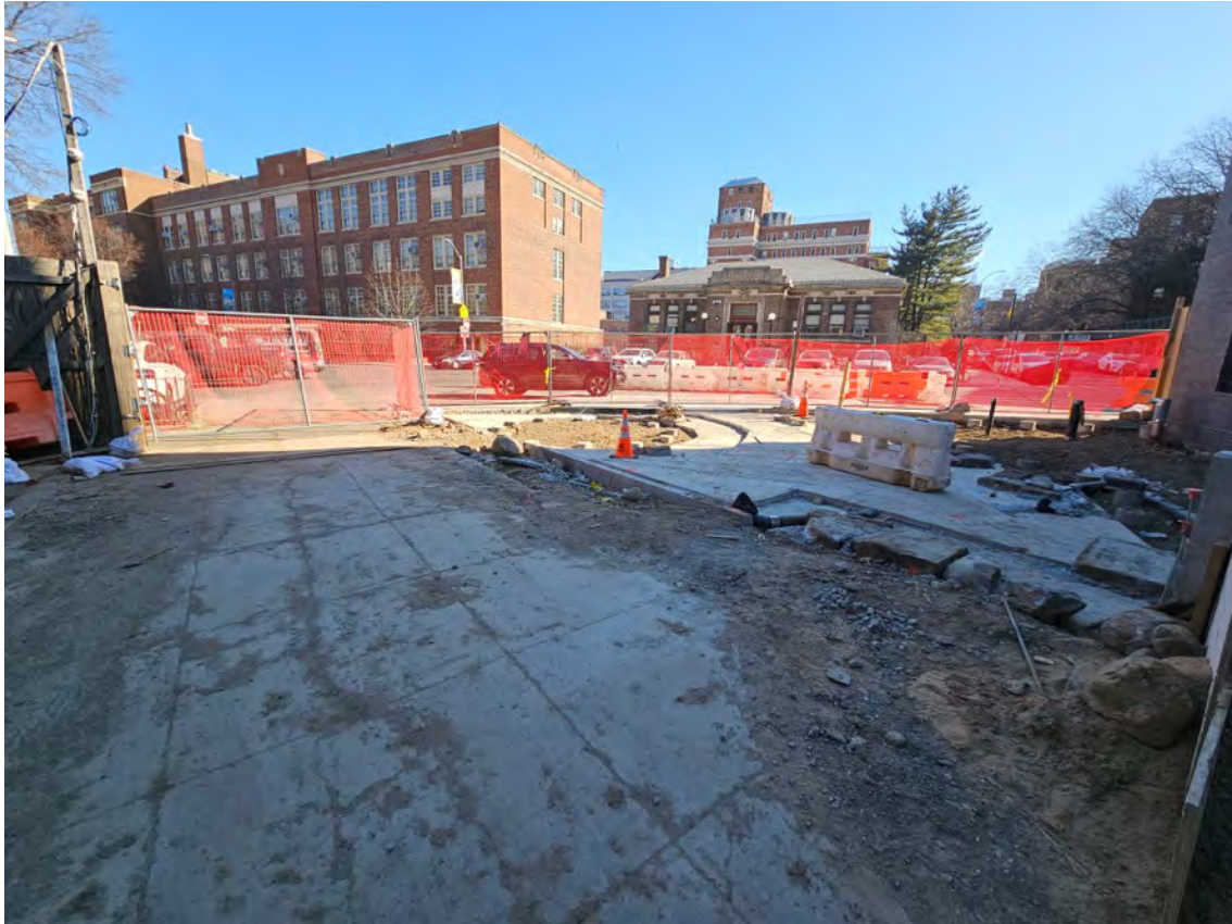
Photograph 5. Area 1, location after excavation and permanent soil capping, view looking northeast.
