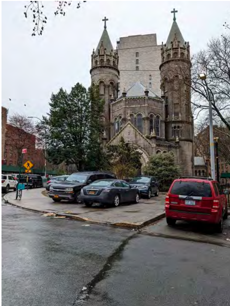
Photograph 1. Area 1 at the northern tip of the project site (raised area with parked cars) prior to excavation, looking southeast from St. Edwards Street and Monument Walk.
