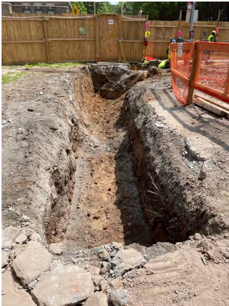
Photograph 14. Area 3, Support of Excavation Trench during archaeological monitoring, view looking east.
