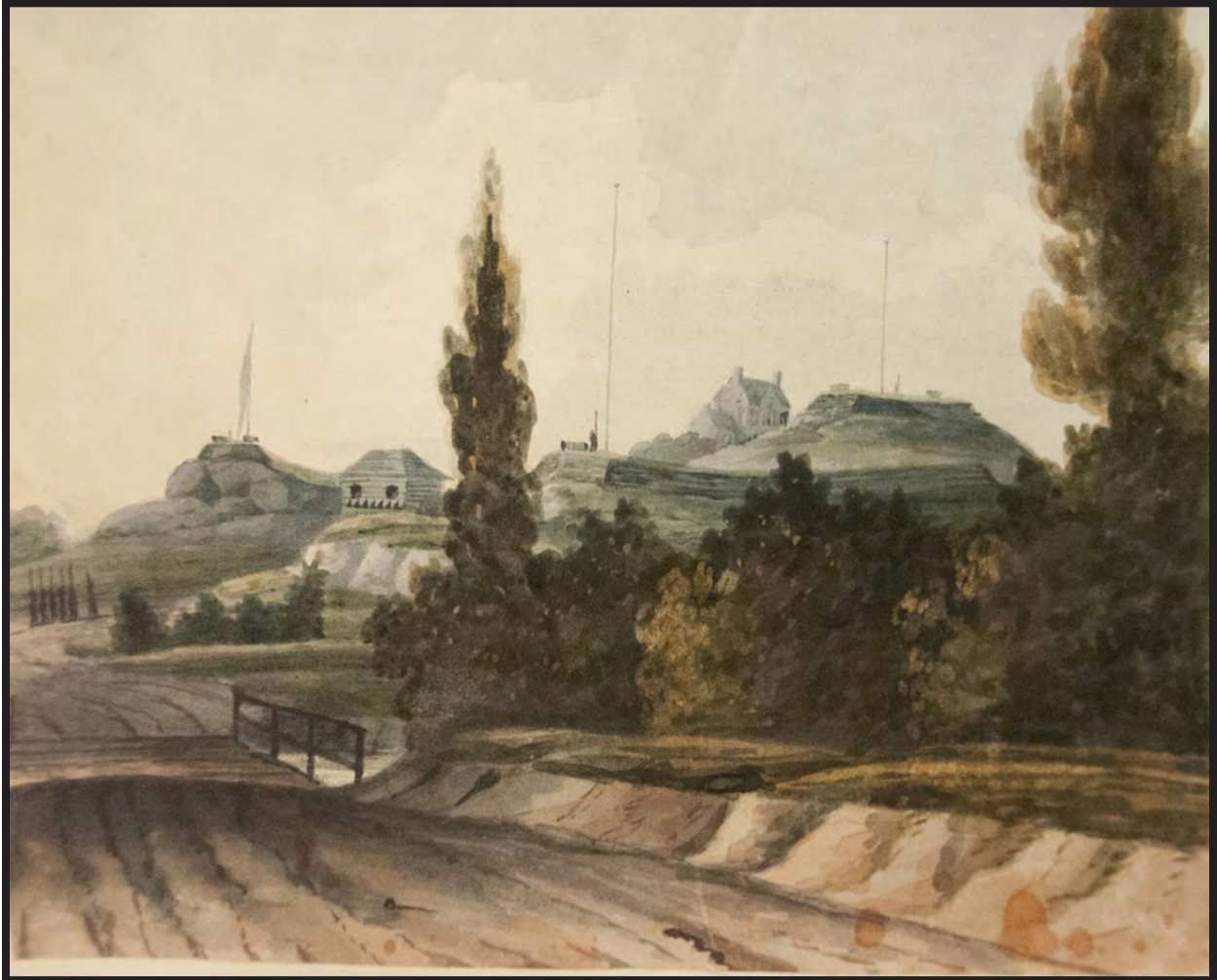
Figure 2.3. John Joseph Holland Associates. Untitled View of Fortifications at McGown's Pass. 1814. This view, looking southeast, shows the Kingsbridge Road in the foreground leading up to the McGown's Pass Gatehouse [592-2], which is flanked by Fort Clinton [591-3] to the left and Nutter's Battery [592-6] to the right. Behind and to the right of Nutter's Battery is Fort Fish [590-13] and beyond and to the left of Fort Fish is the McGown's Tavern property [589-12]. Source: New-York Historical Society, Luce Center, Object No. 1889.23ab.
