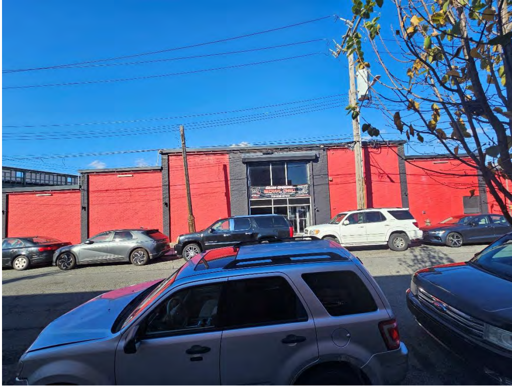
Photograph 3. The main entrance to the Lot 65 Bowl 360 facility on Bouck Court. View looking north.
