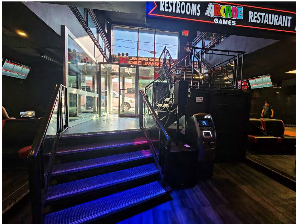
Photograph 7. The main entrance of the Lot 65 Bowl 360 facility from the interior looking south toward Bouck Court. The car in the background is at the street level and the floor in the foreground is the first floor level of the bowling facility.
