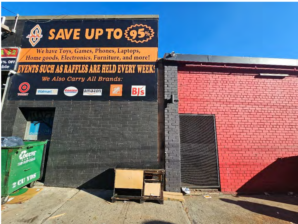
Photograph 2. Detail of the Lot 65 Bowl 360 facility Shell Road emergency exit door on the right, at the sidewalk level. View looking east from Shell Road.
