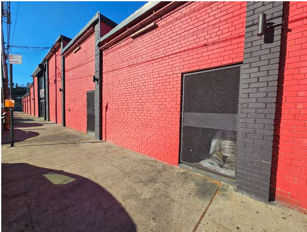
Photograph 4. Detail of the Lot 65 Bowl 360 facility entrances on Bouck Court. The main entrance is in the left background and an emergency exit door is in the left center. View looking northwest.
