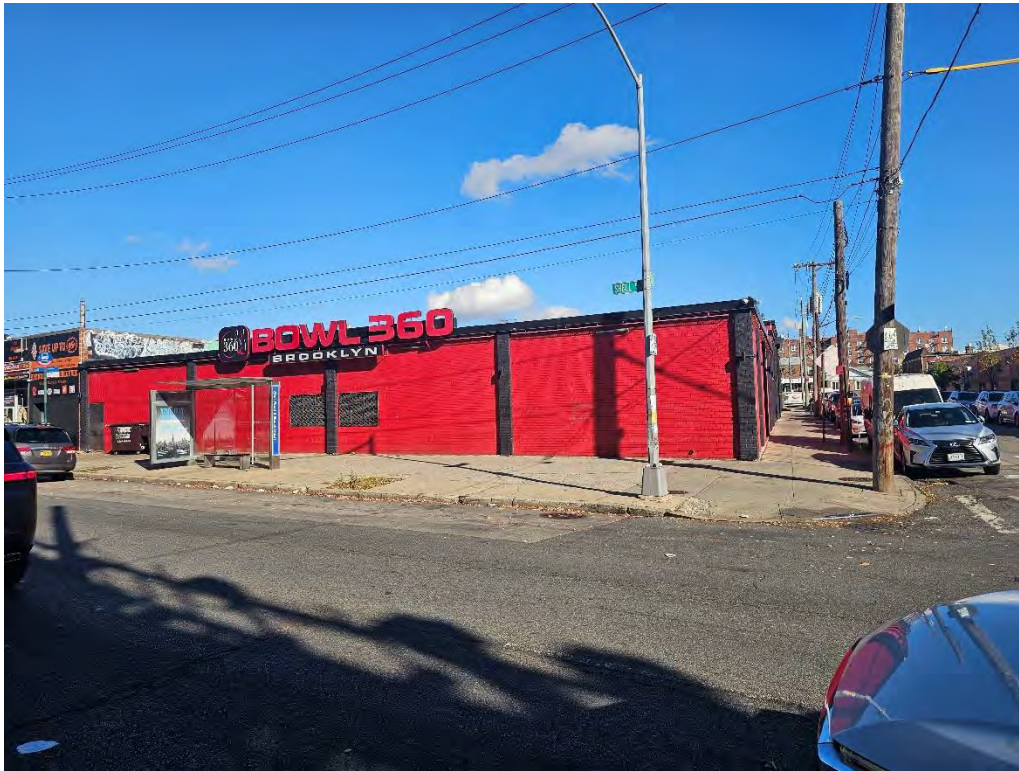
Photograph 1. The Lot 65 project site containing the Bowl 360 facility. View looking northeast from the intersection of Shell Road and Bouck Court.
