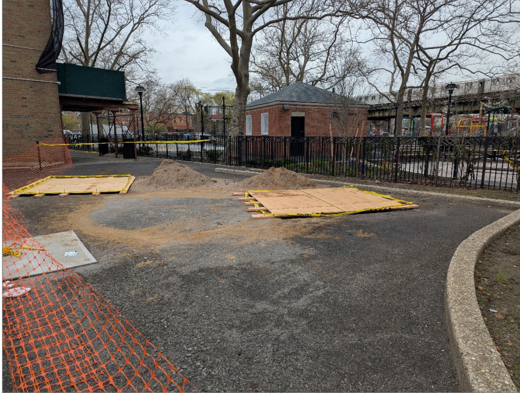
Photo 4. Restoration of the parking lot after Unit backfilling, view to west.
