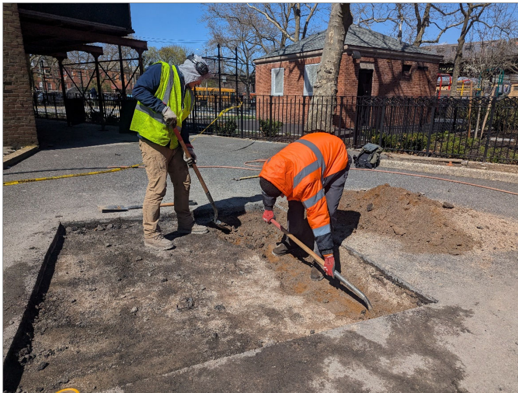
Photo 1. Monitoring of removal of asphalt and subbase by hand, view to northwest.
