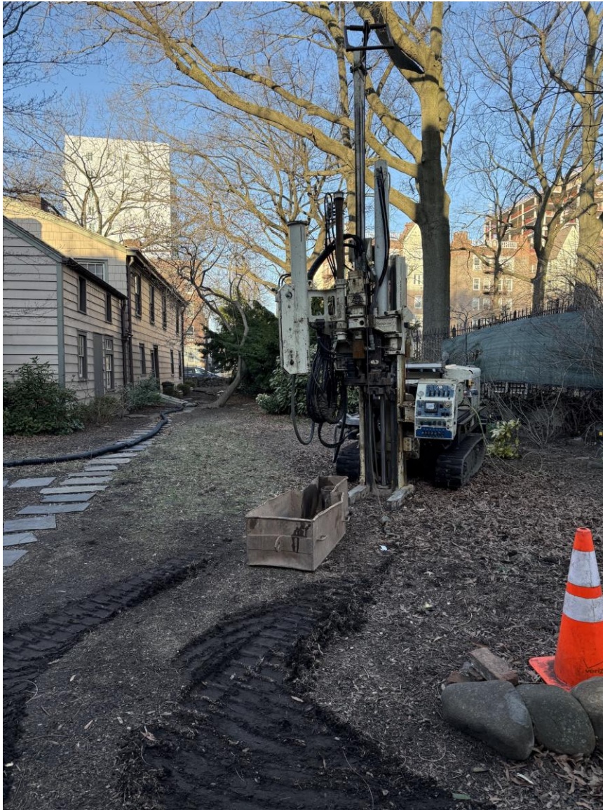
Image 1: Testing location north of the house.
