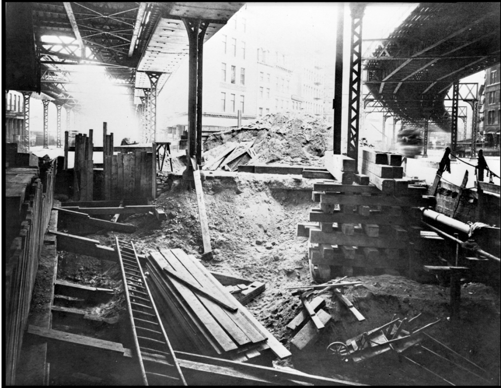
Image 8: Manhattan, Chatham Square excavation, looking south, March 10, 1904 (New York Historical Society).
