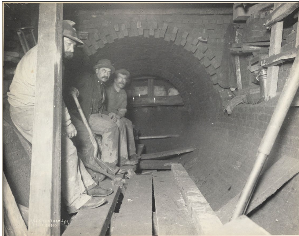
Image 9: Contract One. Underground photograph ca. 1905. Subway Construction Photograph Collection (New York Historical Society).
