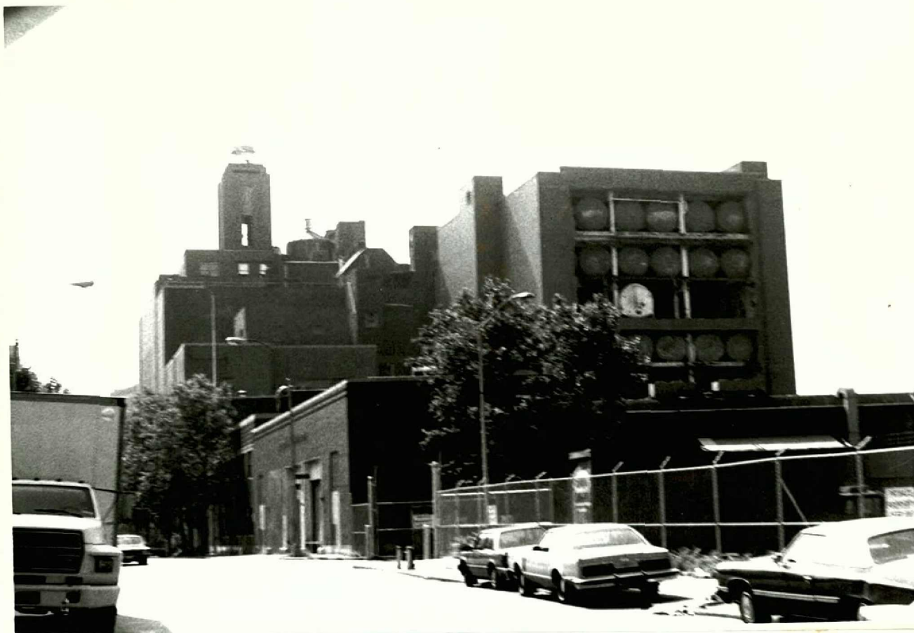
Plate 2. View of Schaefer Brewery complex as seen from the north. Aluminum tanks are visible in the seven story building on the right, from which the north wall has been removed. Kent Avenue runs along the east side of the structures. The East River is immediately to the right of these buildings. View looks south. 20 September 1983.
