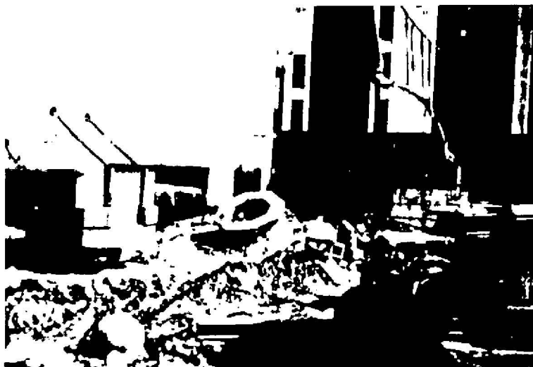
"another view of the site looking north. The con- crete octagon is a tank foundation that has been tipped up by the steam shovel" 1940
