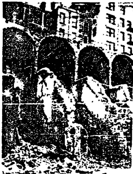
The rear of the century-old warehouses which have been demolished, showing the arched roof and eight-foot-thick walls. The rear wall was slanted and served as the retaining wall for the houses above. These houses, facing Columbia Heights, will not be demolished.
