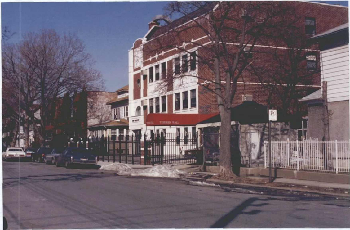
Plate 1a Yeshiva Teferes Yisrael Existing Building View Northeast from Corner of East 35th Street and Avenue L
