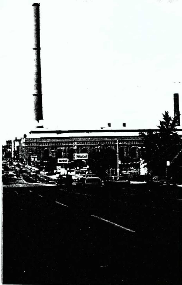
Plate 2. Looking south from 65th Street and West End Avenue. Note Mobil Station at 61st Street and Con Edison Plant at 59th Street (photo: 6/25/86).
