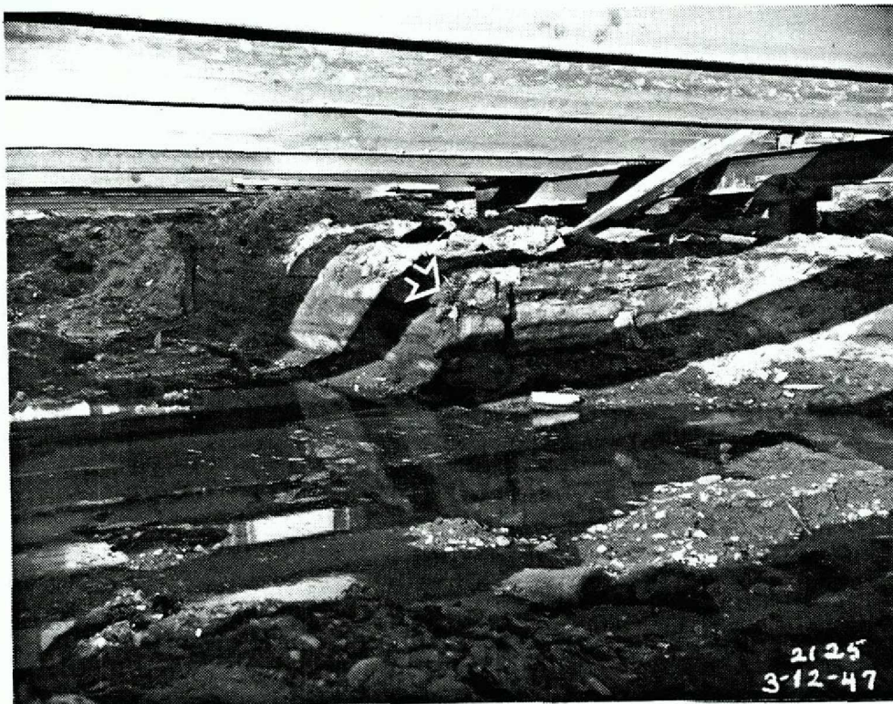
Plate 10. Log cribbing partially exposed in the southwestern segment of the blower building site, about 60 ft. north of Battery Place (the southwestern corner of this construction is indicated by an arrow). Possibly a wharf on Thomas Farmer's water lot, it is not documented in any known record or on any known map (TBTA 3/12/47).
