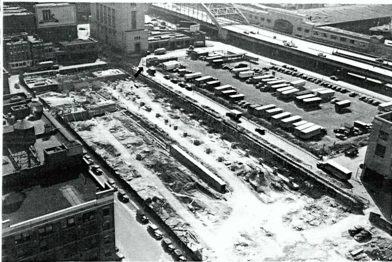
42 Site B during foundation excavations (9/12/47) looking south from near Charlton Street. Columns on west side of site are in place. Note Site A, a parking lot, and the produce distribution platform and building in Figure 39 is now a diner (arrow). (Photo courtesy of NY-NJ Port Authority TT-515)
