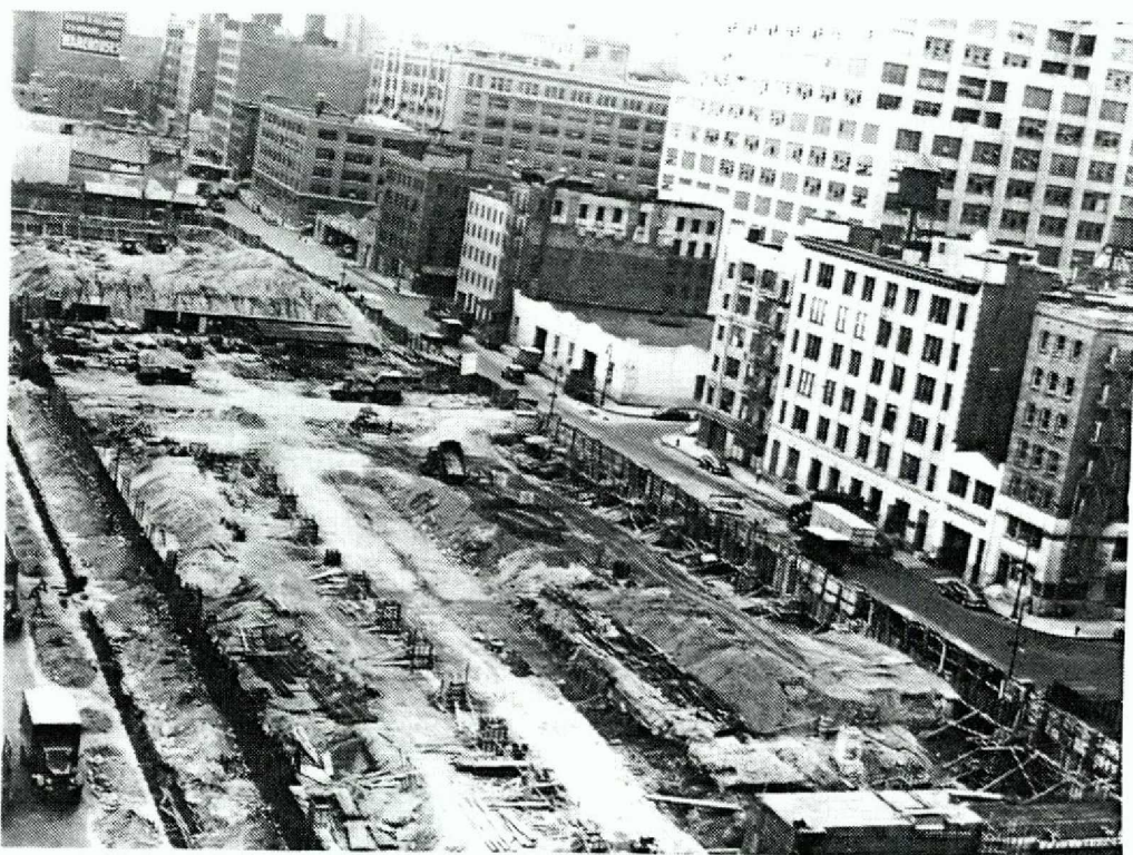
41 Site B during foundation excavations for the Union Terminal Building, looking north from Spring Street (8/21/47). Note that columns on western part of site are in place, those to the east still have to be excavated. Also note depth of excavations along the property line on Greenwich Street to the right. (Photo courtesy of the NY-NJ Port Authority TT-499)
