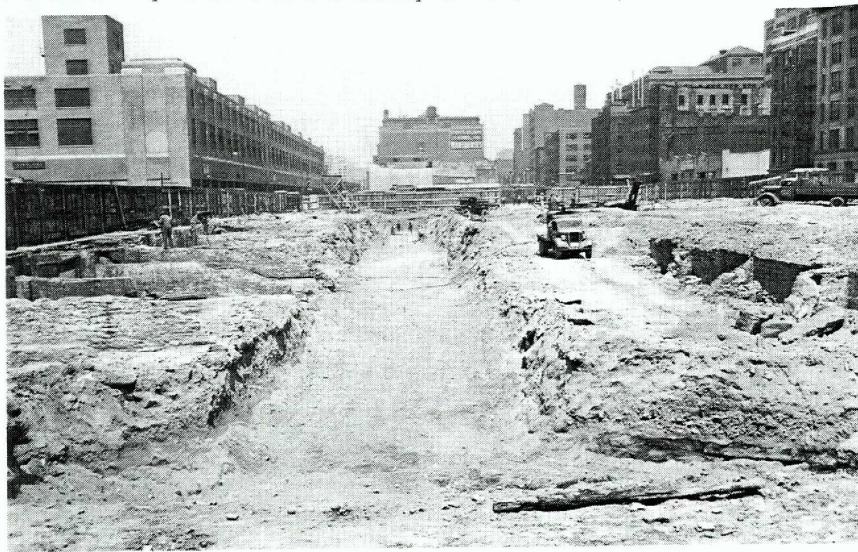
40 Same as above, May, 1947, beginning of excavations (column line is in center of photo). Note old building foundations and the St. John's Park Freight Terminal (now the St. Johns Building) to left rear. (Photo courtesy of NY-NJ Port Authority (TT 406)
