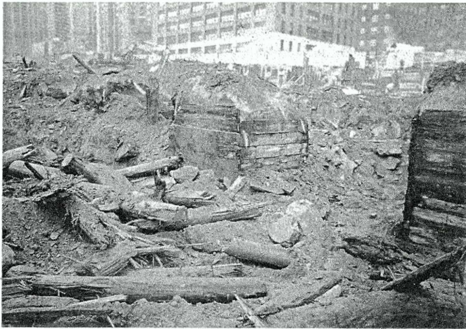
8 Concrete foundation columns in wooden forms were found throughout the site (arrow). Similar constructions destroyed the eastern end of the southern wall of Block 1 and the southern end of the unmortared western long wall of Block 2. Note wooden logs, probably former pilings or possibly wharves. View is northeast toward W 63 St and West End Ave. (Geismar 2/21/94)
