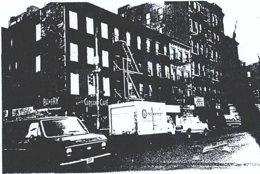
Plate 17. View of buildings in the project area at the southeast corner of Ninth Avenue and 39th Street.
