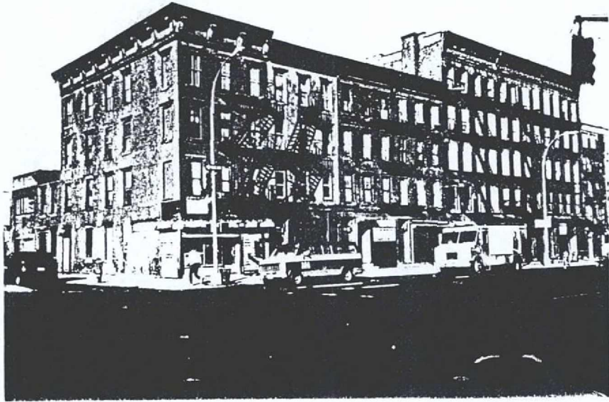
Plate 11. View of buildings in the project area at the northwest corner of Ninth Avenue and 37th Street.
