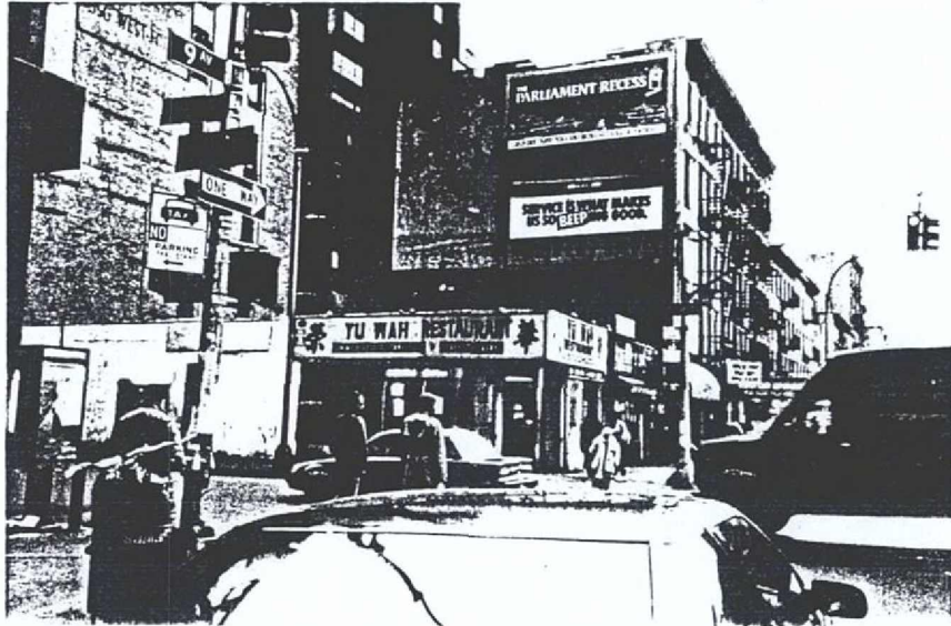
Plate 23. View of buildings in the project area at the southeast corner of Ninth Avenue and 40th Street.
