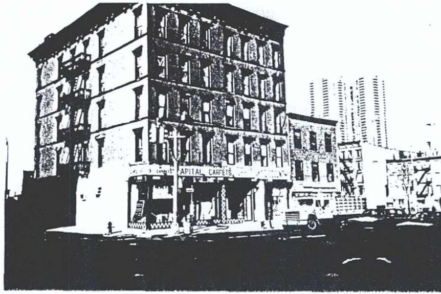
Plate 15. View of buildings in the project area at the northwest corner of Ninth Avenue and 38th Street.
