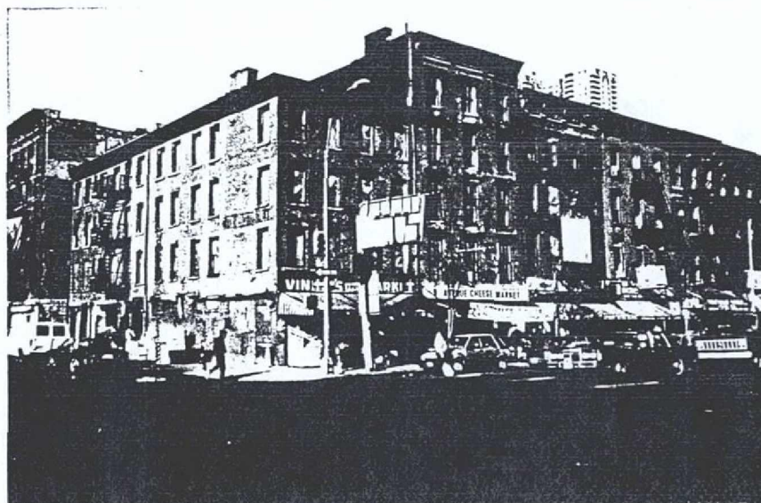
Plate 20. View of buildings in the project area at the northwest corner of Ninth Avenue and 39th Street.
