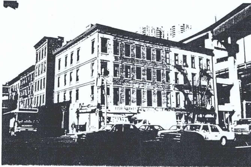
Plate 22. View of buildings in the project area at the northwest corner of Ninth Avenue and 40th Street.
