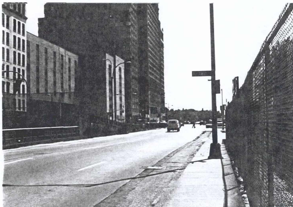
6. Project Area looking south from intersection of Rector and West Streets
