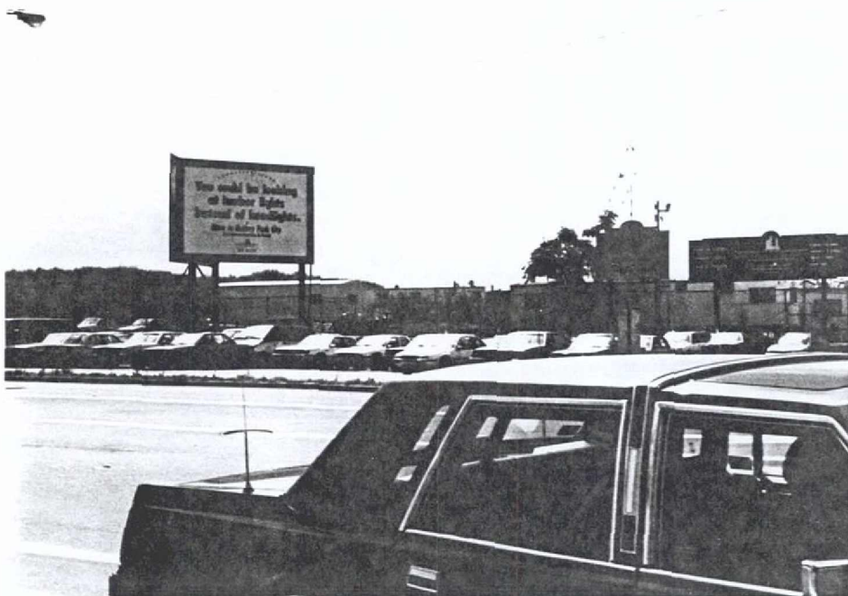
4. Project Area looking southwest from Brooklyn-Battery Tunnel Entrance
