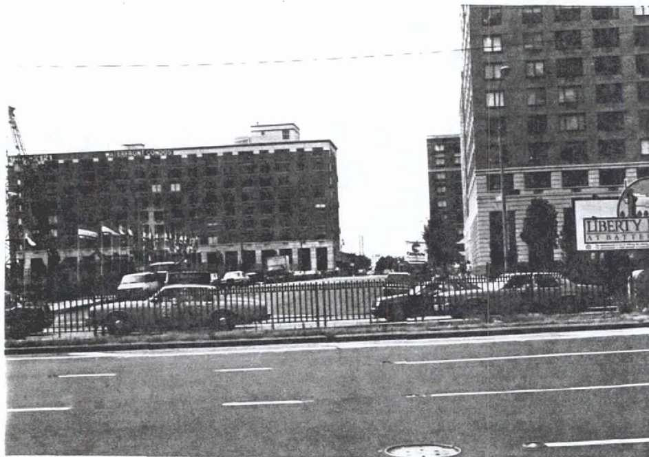
5. Northern boundary of Project Area looking west toward West Thames Street
