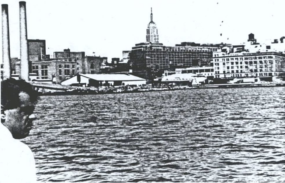
Gansevoort Plant, Storage Shed, Bulkhead View from the Hudson River facing northeast 4/27/89
