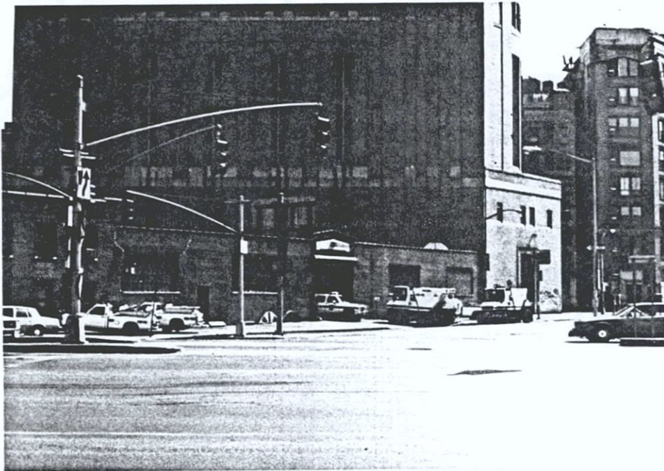
Canal Street, Base of Holland Tunnel ventilator building, city parking garage Facing east from Marginal Street between Piers 32 and 34 9/13/89
