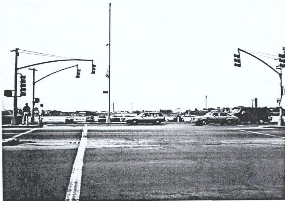
West Street, Marginal Street Typical view at intersections of cross streets. Facing west from West 12th Street 9/13/89
