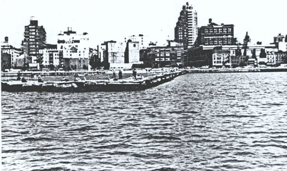
Pier 46, Bulkhead The public now use Pier 46 as recreational space. View from the Hudson River facing east 4/27/89
