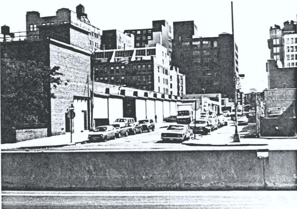
Leroy Street Facing east from Marginal Street 9/13/89
