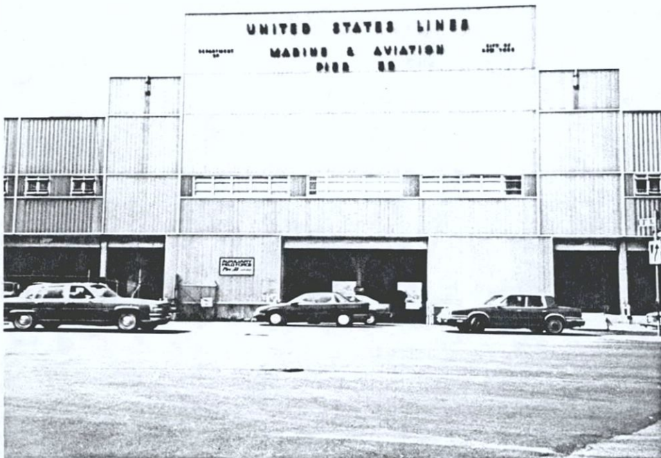
Pier 59 piershed Facing east from West 18th Street 9/13/89
