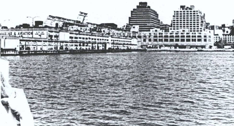
Pier 40 complex, Bulkhead, St. Johns Building View from the Hudson River facing northeast 9/13/89
