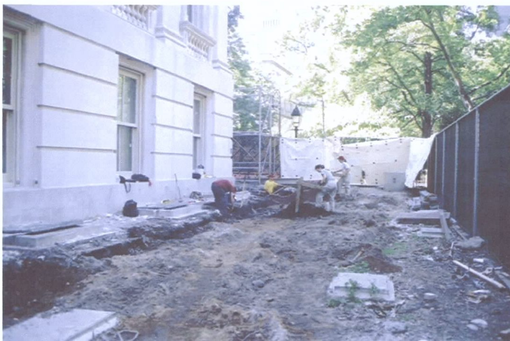
Photo 9. View south of excavations along the east side of the courthouse.
