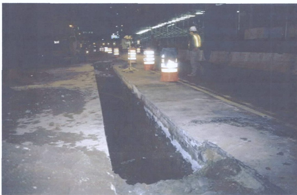
Photo 7. View east of Trench 1, west bound lane of Chambers Street.
