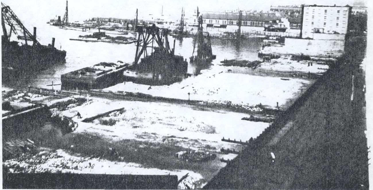
FIGURE 71. Dredging for Gansevoort Piers between Bank and Gansevoort streets, 1897-98. West Street is at the right and the West Washington Market is in the background (Collection of South Street Seaport Museum).
