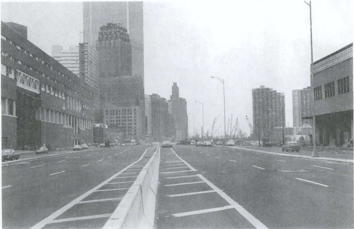
FIGURE 98. View of Lower West Street (Area 2 in Figure 3), looking generally southward from North Moore Street. The piers are at the right, the cranes in the distance mark the construction site of Battery Park City, and the World Trade Center is visible extending off-camera top left. (Michael Spozarsky, photographer, April 1983.)
