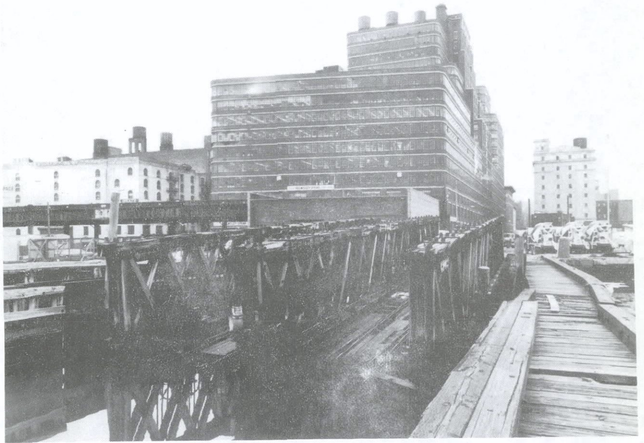
FIGURE 81. View eastward at Baltimore & Ohio Railroad float bridges, W. 26th Street (Michael Spozarsky, photographer, 1980).
