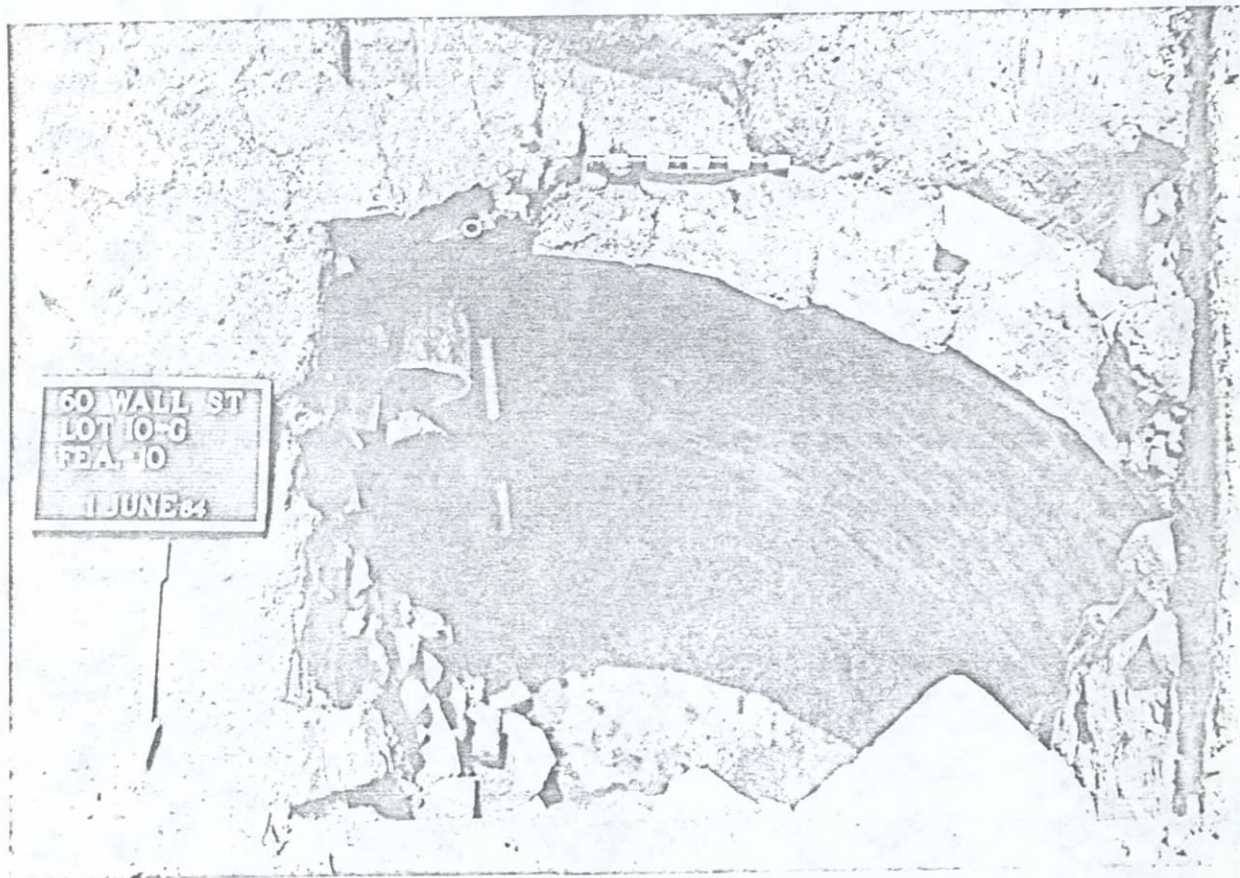
FIGURE 65. View southward of southwest quadrant of interior of Feature 10, brick cistern. Note the end of a lead pipe (Feature 26) extending through the feature's south wall (left of center in photograph). (Photographer: Tony Masso, 1984.)
