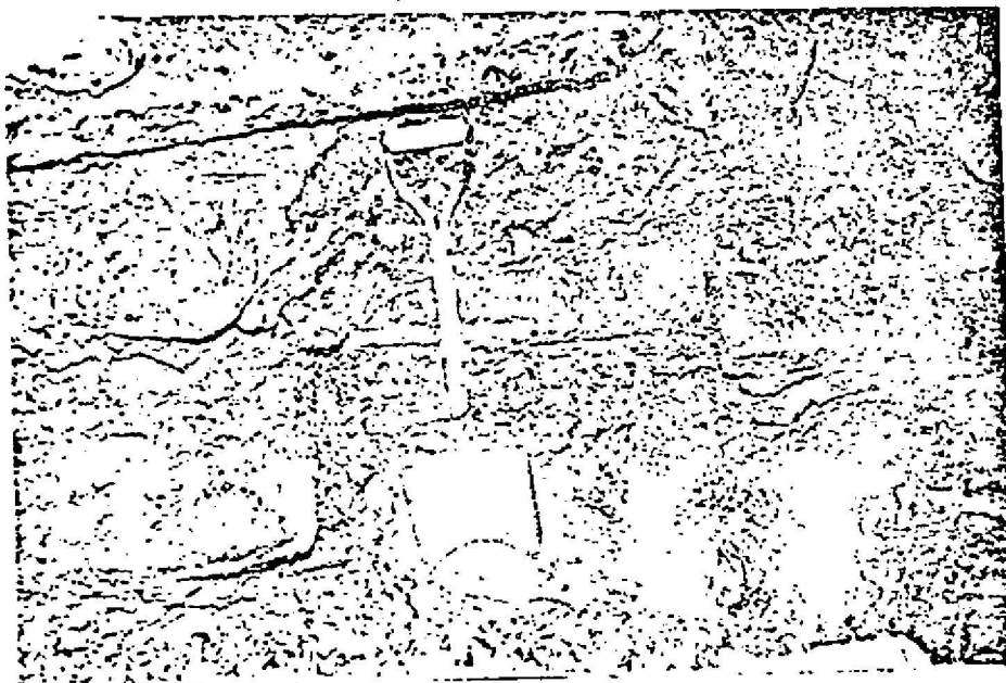
Here the uneven lengths of the spread-footer planks under the south wall of the building at 189 Front St. are clearly visible (Sch 9, x 14, looking S)
