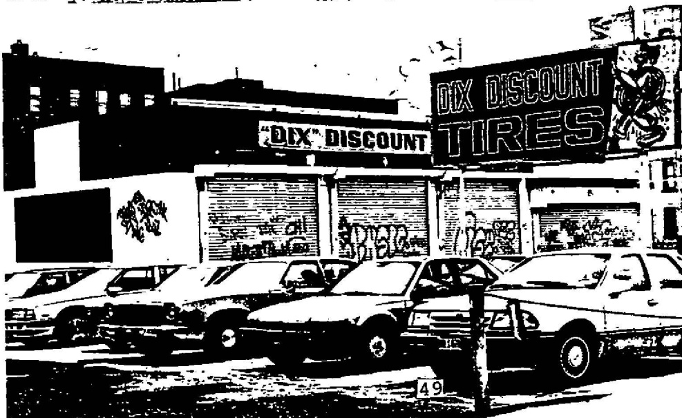
Looking southeast from Broadway at service station structure on Lot 7, Block 2234 Project Site on the left
