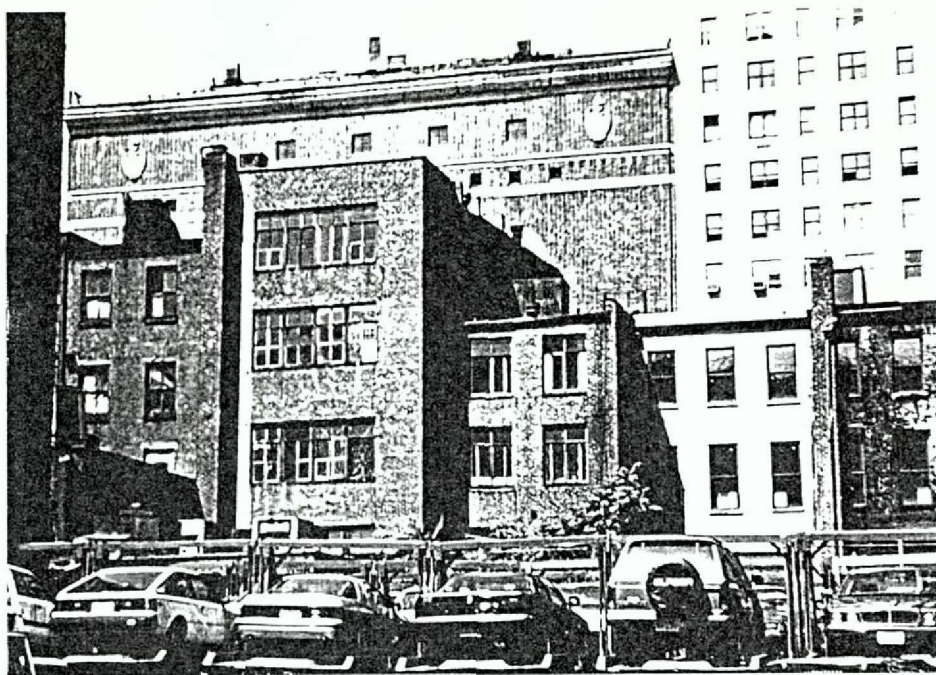
Photo 5: From 33rd Street facing north toward 34th Street. Showing, from right to left, the rears of #304, 306, 308, 310, & 312 34th Street.
