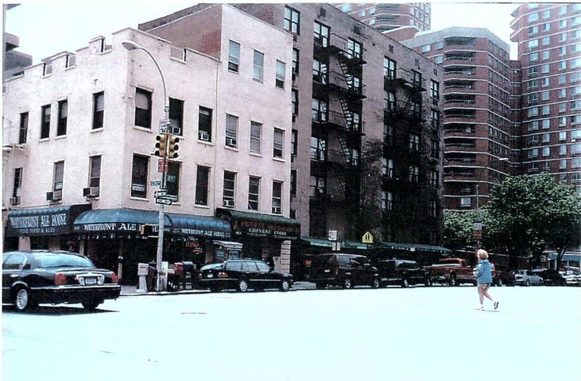
Photograph 12: Southeast corner of Second Avenue and East 30 th Street (Block 935). Second Avenue Between East 31 st and East 29 th Streets.
