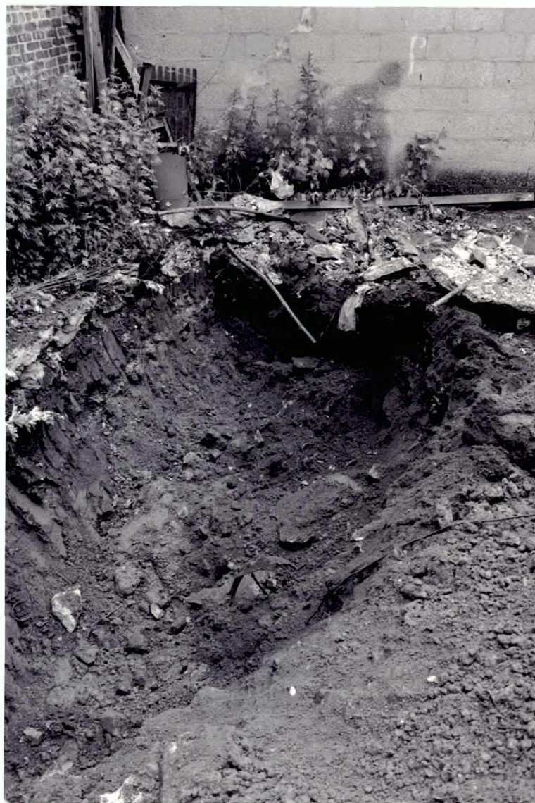
Plate 4 View of Backhoe Trench 5 looking north.
