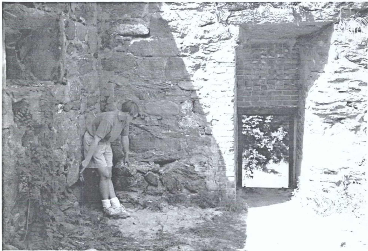
Plate 5.5. Blockhouse [809-2]: view of interior looking west southwest at the southwest corner; figure is pointing at the location of the original entrance, to her right, and to the foundation offset, possibly used to support floor joists, to her left (Photographer: Richard Hunter, August 1990).
