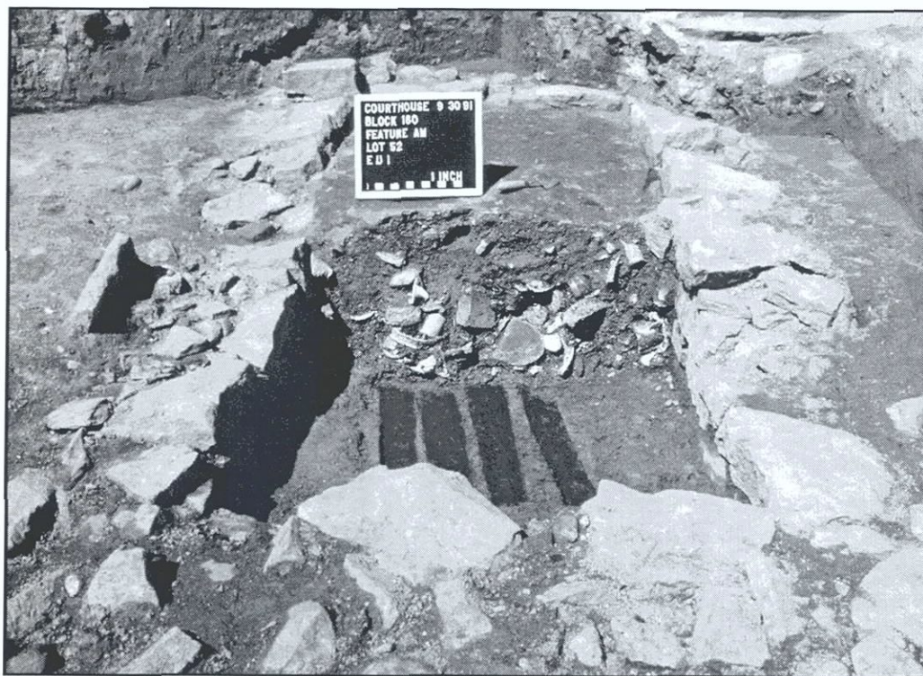
Figure 58. Feature AM, Lot 52. Sandstone foundation and floorboards for icehouse behind Conlon's oyster cellar.
