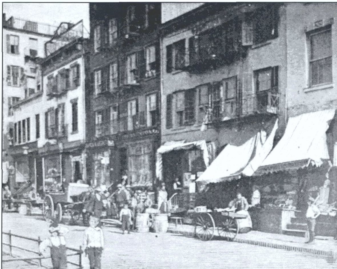
Figure 32. Pearl Street (left to right, 470 through 464) in the early twentieth century. Courtesy of the New York Public Library, Astor, Lenox and Tilden Foundations.
