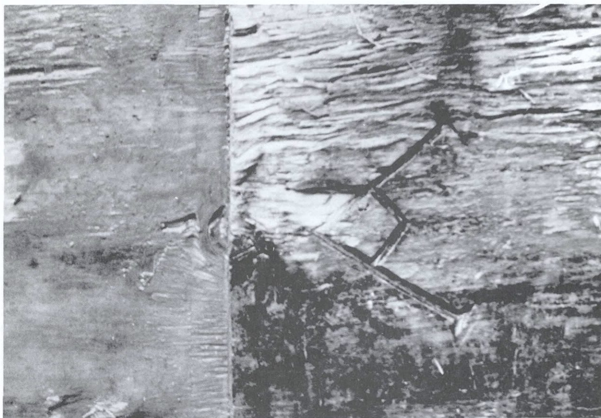
PLATE 4.6 Close-Up of Mark on Reused Mast
