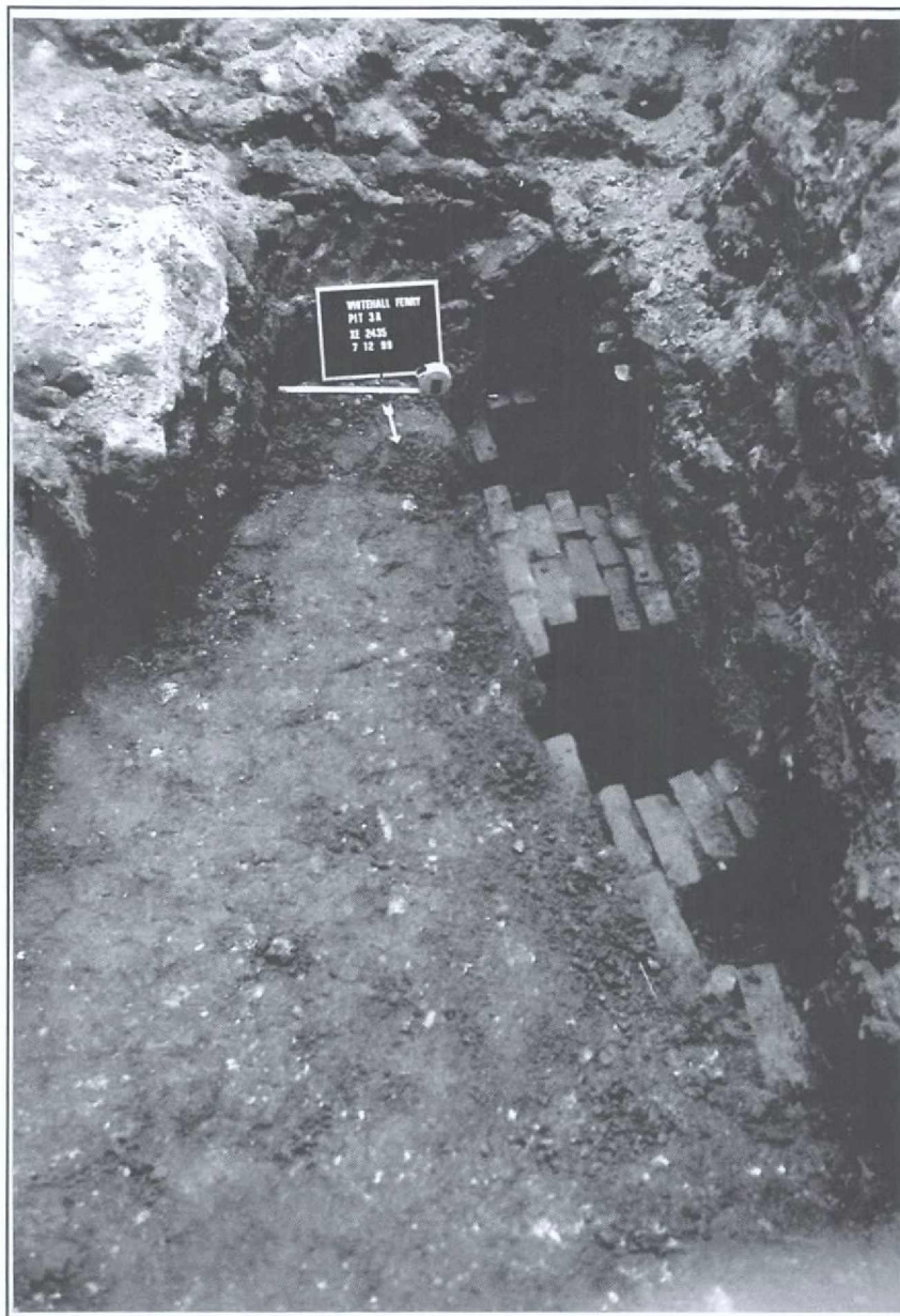
PLATE 7: Test Pit 3A at a Depth of Approximately 5.5 Feet Below Grade, Showing Top of Abandoned Brick Sewer. Scale is 1 Foot Long. View to South.
