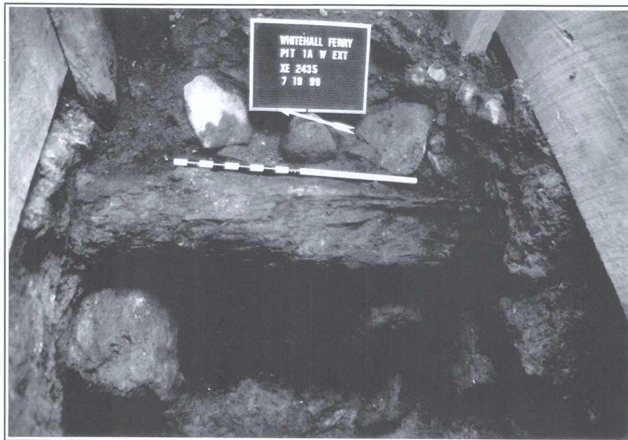
PLATE 5: Feature 1 in Test Pit 1A Extension at Depths of 4.8 to 7.0 Feet Below Grade, Showing Western Edge of Timber-Built Landfill Retaining Structure. Scale is 2 Feet Long. View to East.
