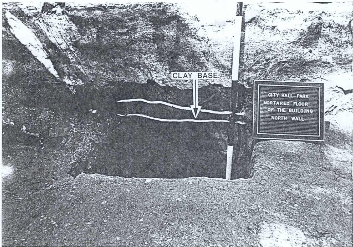
Figure 2:6 Interior foundation wall. The clay base underneath the floor also extends under the brownstone foundation. The interior surface of the foundation wall is whitewashed (Photo: Sherene Baugher).
