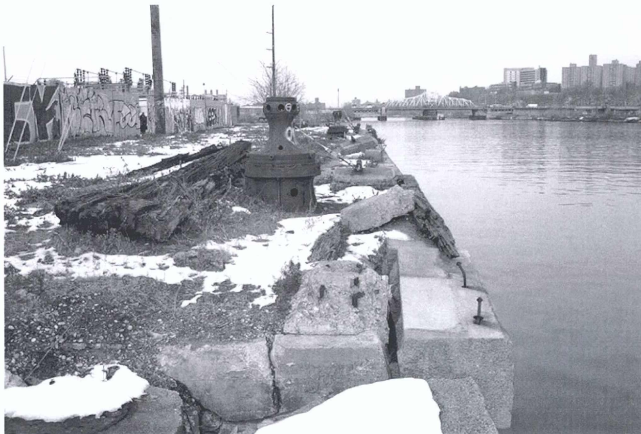
Figure 4.10. Concrete bulkhead docking area with iron mooring posts north of the APE, facing northeast. Sherman Creek Ecosystem Restoration Project, New York County, New York (PCI 2002).
