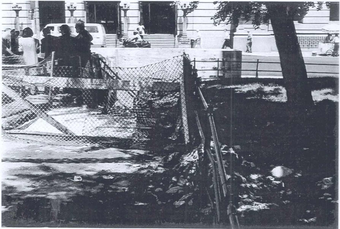
Figure 1.4 CHP/2 Site in June 1992, during the installation of public lavatories designed by J. C. Decaux.
