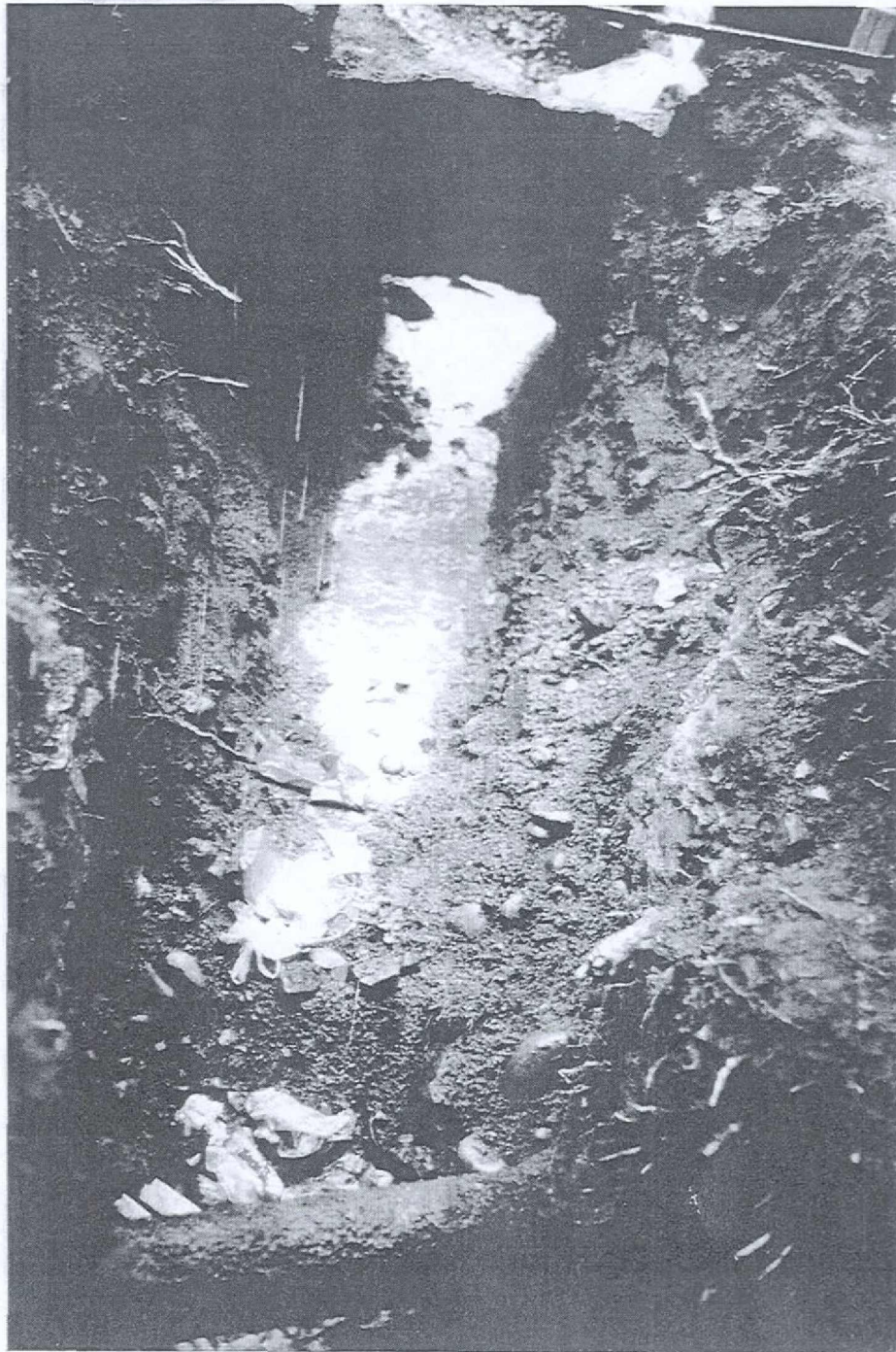
Figure 1.6 CHP/2 Site in June 1992 during the installation of public lavatories designed by J. C. Decaux: east-west construction trench.
