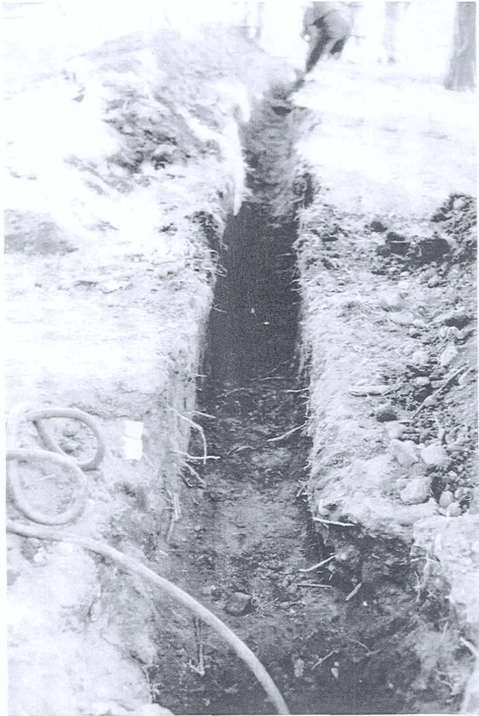
Figure 2.5 Second east-west water line construction trench.
