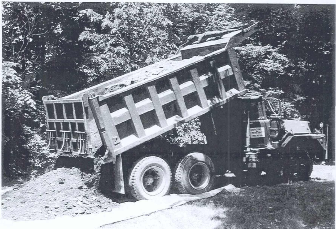
Figure 4.2 Delivery of back-fill soil from the CHP/2 Site to the New Jersey headquarters of Historic Conservation and Site Interpretation, Inc.
