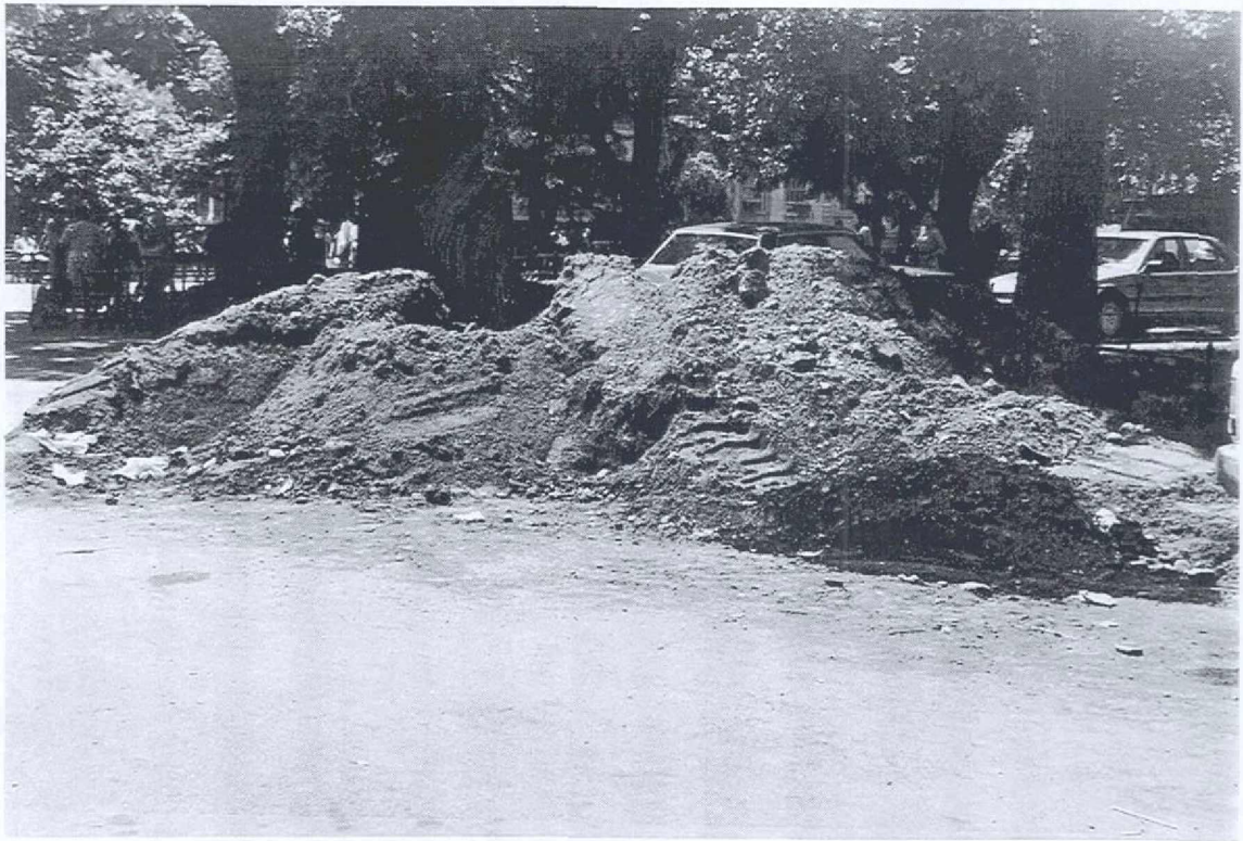
Figure 4.1 Back-fill soil removed from the CHP/2 Site for sifting.
