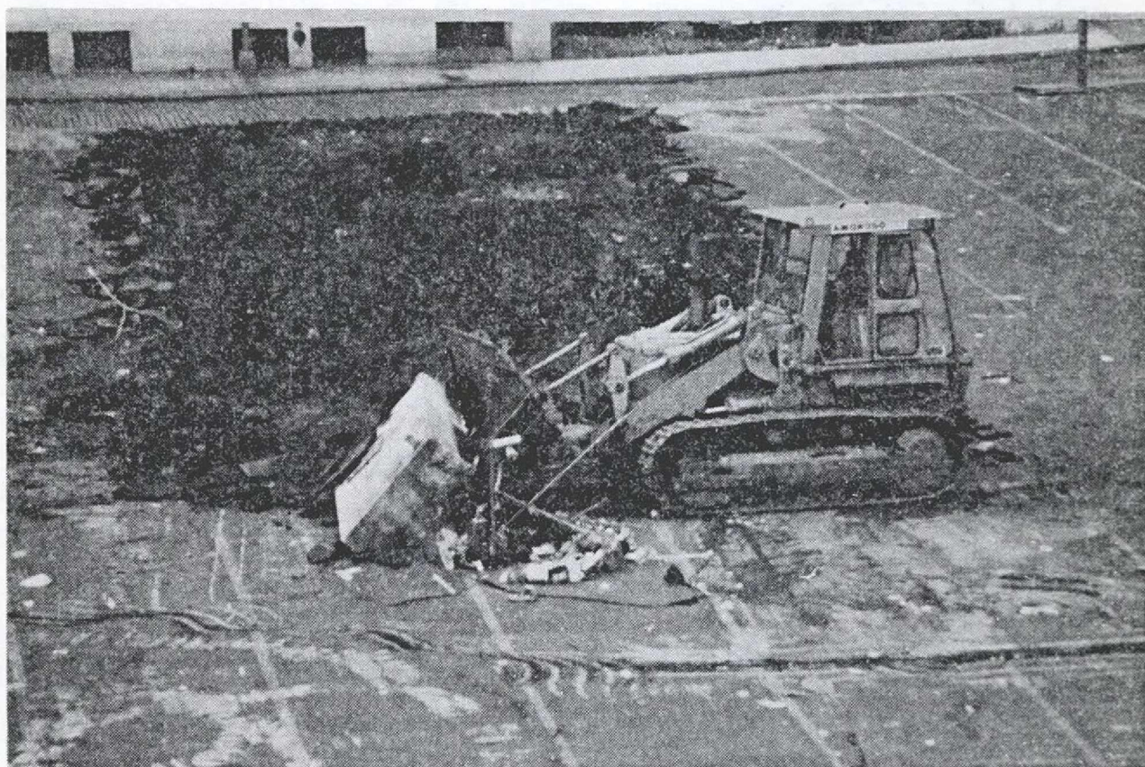
PLATE 1. Parking lot surface broken by a 977 loader and operator in preparation for archaeological investigation of the 175 Water Street block (Block 71). Asphalt removal begun on October 28, 1981.
