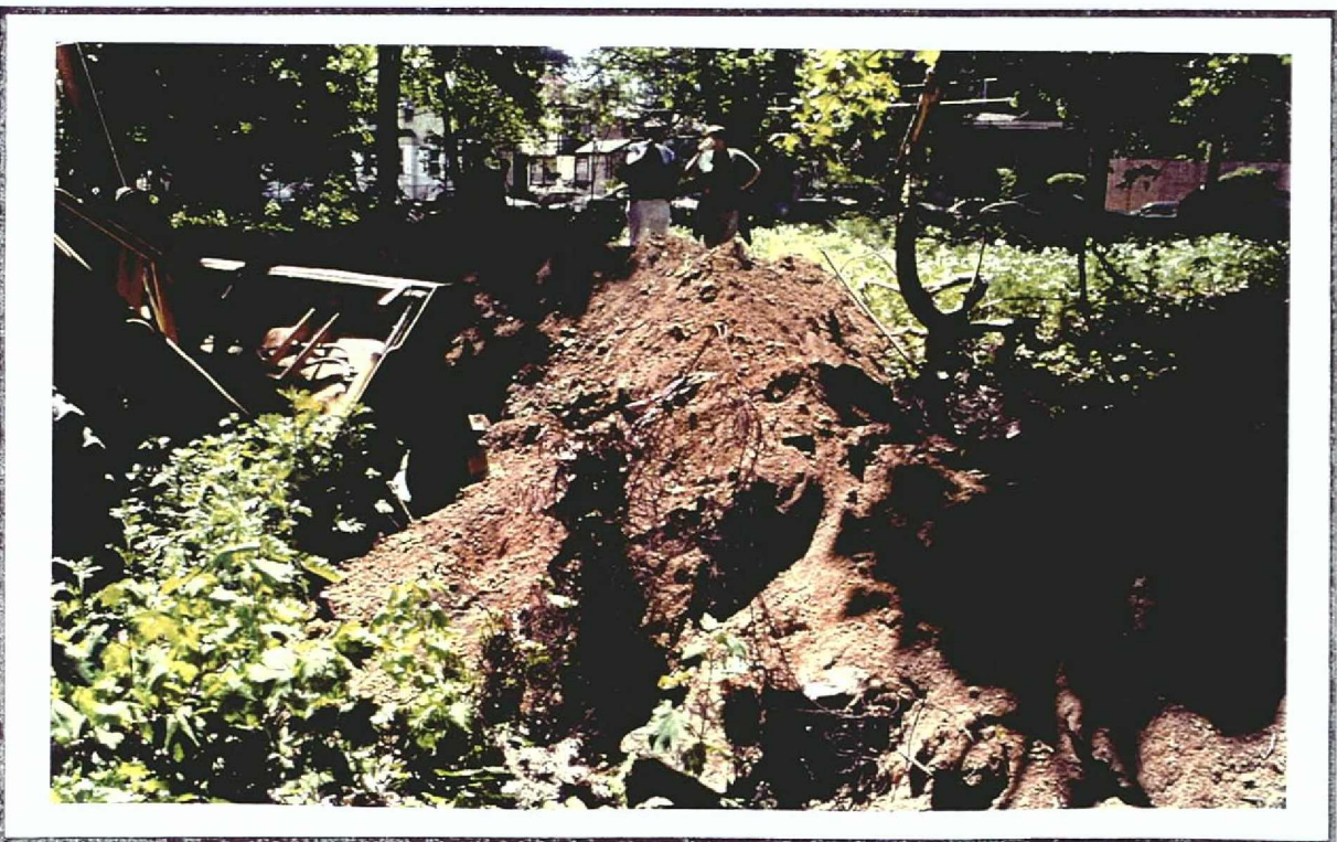
Photo 18: Mechanical trenching on Lot 8 revealed urban soils underlain by soft sandy fill.
