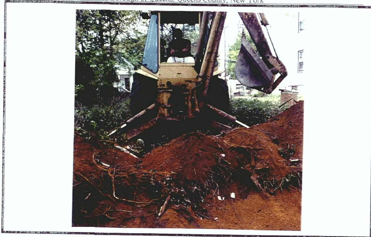
Photo 21: Backfilling on Lot 23 proceeded rapidly, as the soft sand provided no resistance to the backhoe.
