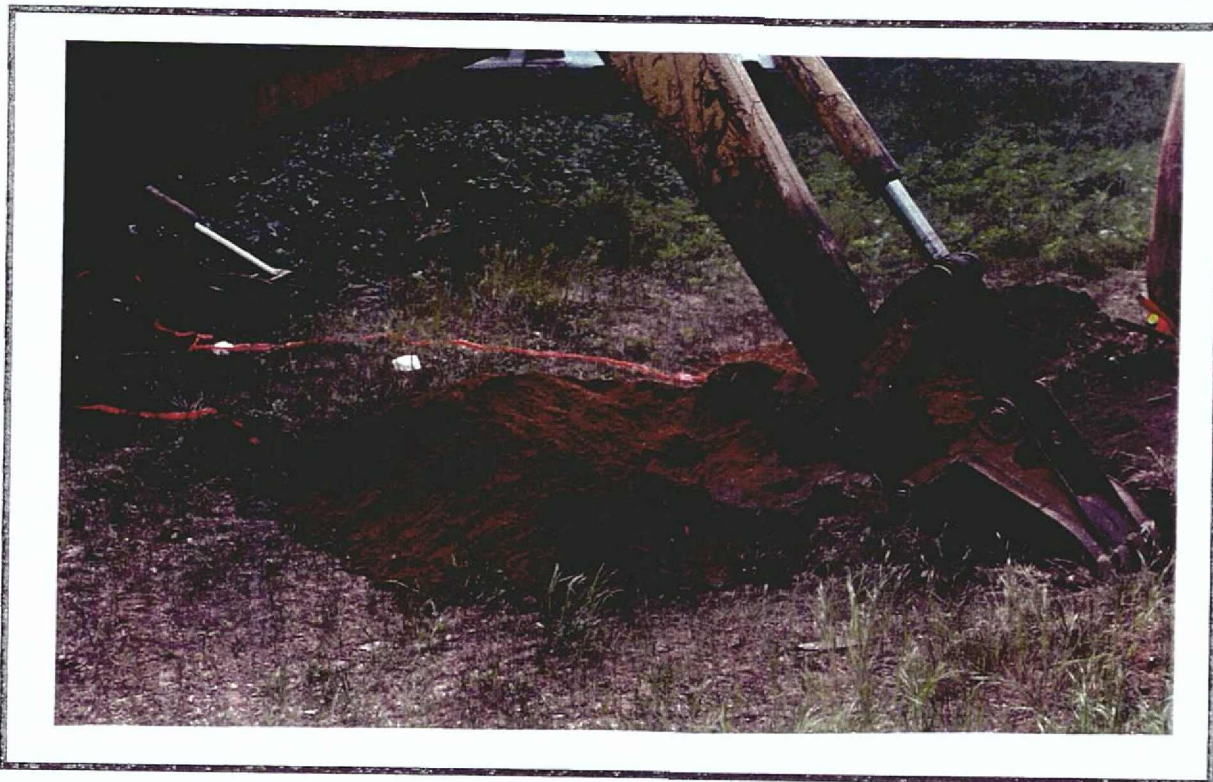
Photo 19: Very dark yellow-orange sandy fill was encountered as soon as the backhoe operator broke the surface on Lot 23.
