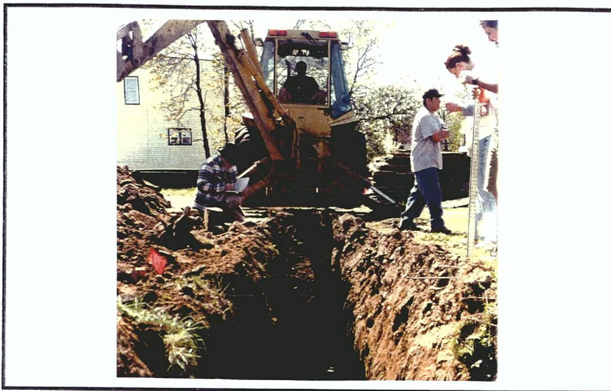
Photo 5: Trench #1 on Lots 11 and 13 exhibitd urban soils mixed with demolition debris to 10 feet below surface.
