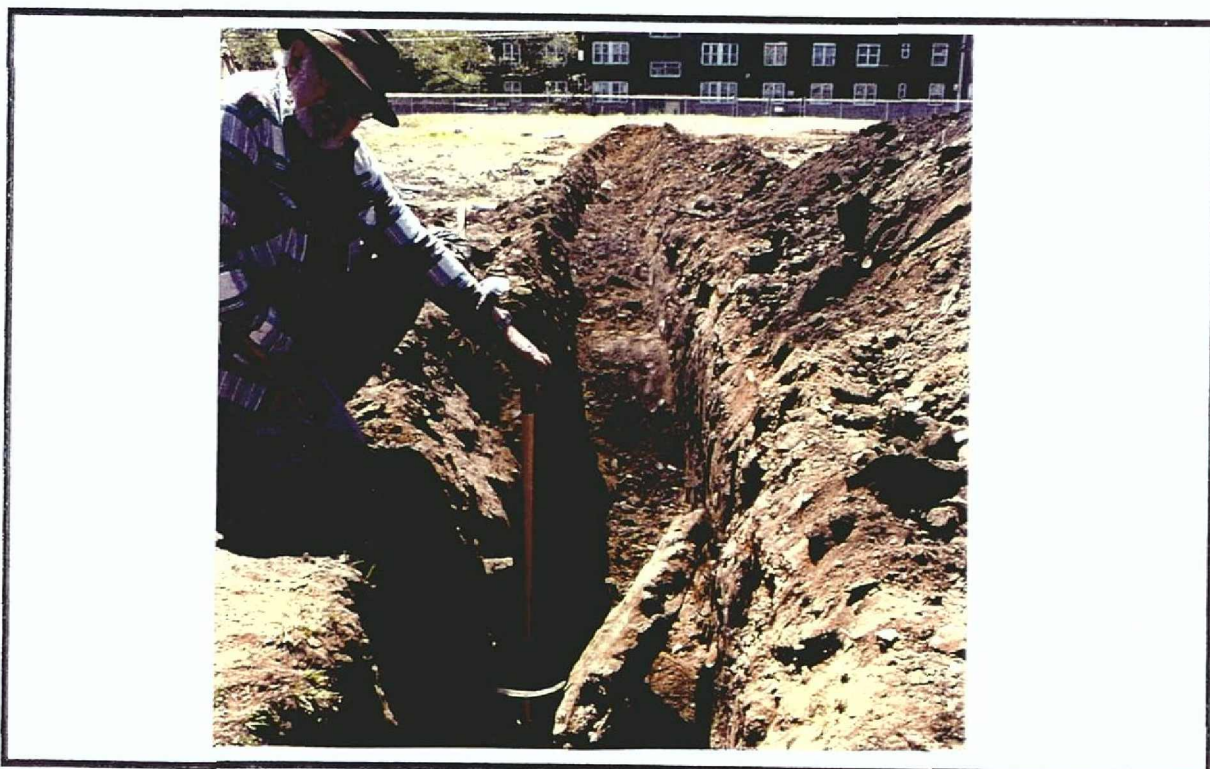
Photo 2: Backhoe trenching on Lot 11 encountered resistance at around 3' below surface. Hand excavation revealed the surface of an asphalt driveway.
