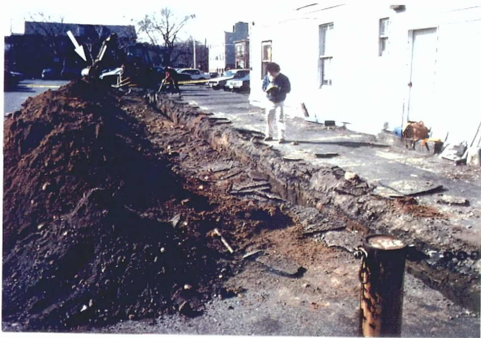
2 Test Trench 1 (TT1) looking southwest from near Hoffman Dr. 58-02 Hoffman Dr., located at the corner of 58th Ave., is to the right. The parking lot for St. John's Hospital extends beyond the test area. The backhoe used to dig the trench can be seen in the background (arrow).
