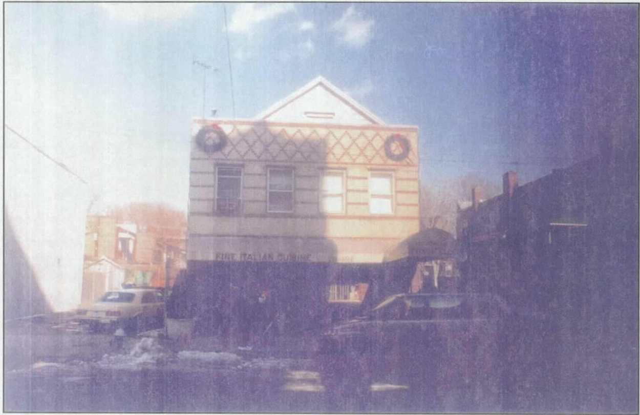
Plate 1: View of Project Area looking northeast across Broadway. The two story structure in the center of photo (46-11 Broadway) is currently a restaurant. The gable-front frame building at the core of the restaurant complex was constructed between 1891 and 1898 (see Figures 8 and 9). The maximum proposed development would result in single story additions in the vacant lots on both sides of the current structure.
