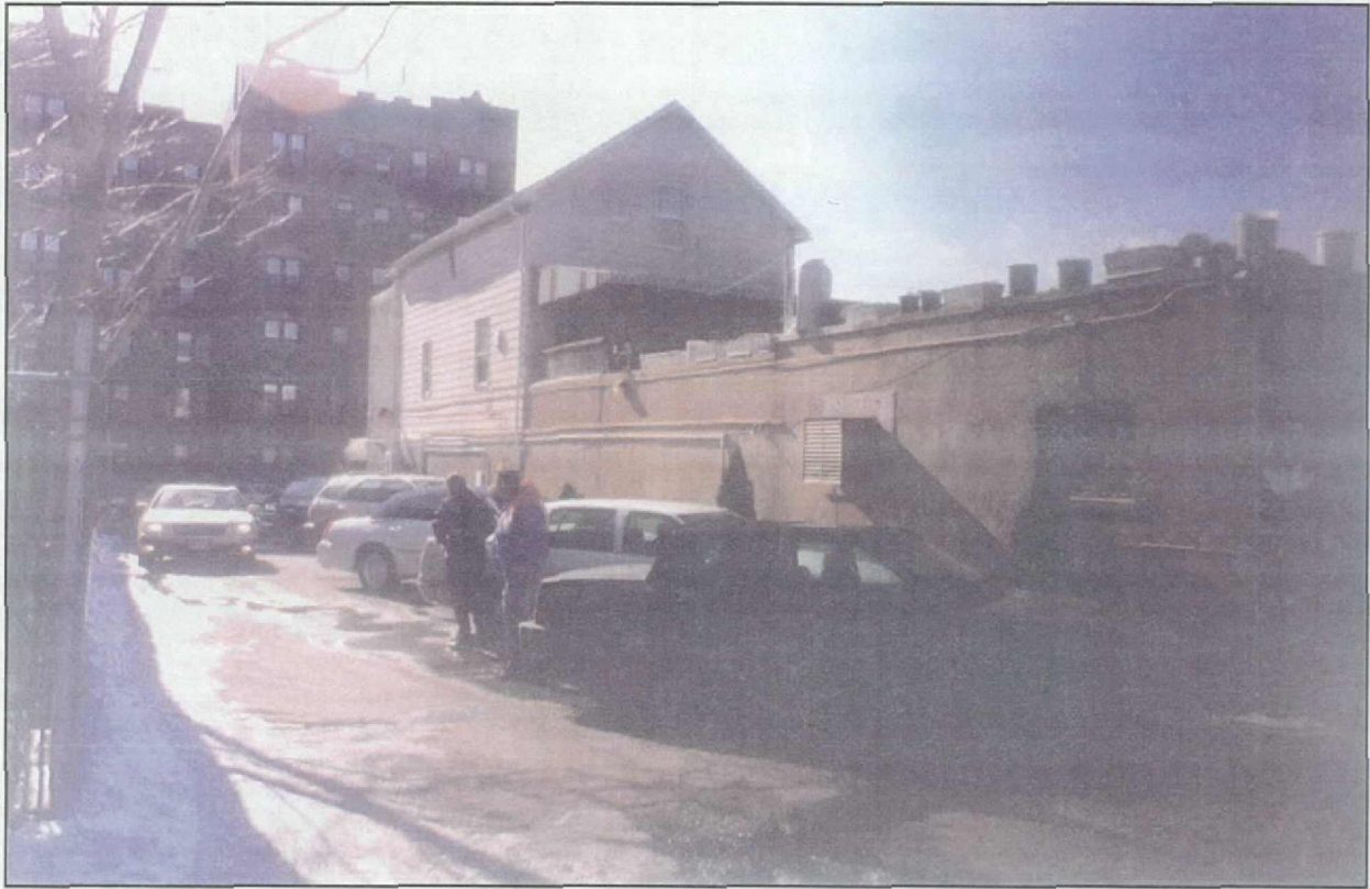
Plate 3. View of the eastern portion of the Project Area (formerly Lot 3) looking southwest toward Broadway. This lot currently has asphalt paving and serves as parking lot for the restaurant. The restaurant (46-11 Broadway) is visible on the right side of photo. Historical research indicates that a small frame structure existed on the rear of this property circa 1891 (see Figure 8); this structure was demolished prior to 1898 (see Figure 9). By 1936 a frame store was present on the front of the property and a garage had been constructed on the rear portion of the lot (see Figure 11).
