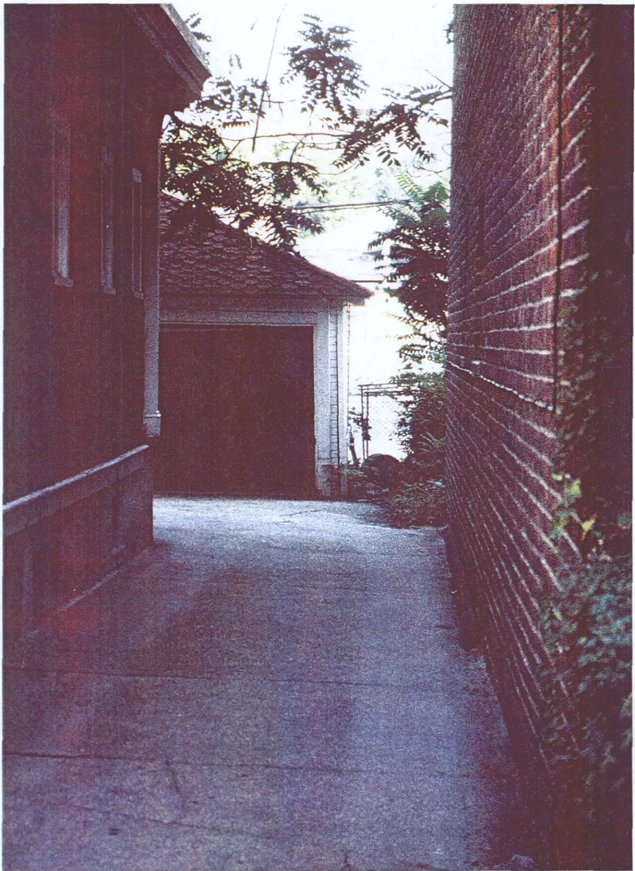
Figure 27. View of east side of Lot 86 2 1/2 story Church structure looking north from pavement on 37th Avenue. Note cement driveway from foundation of structure to lot line of adjacent brick building.
