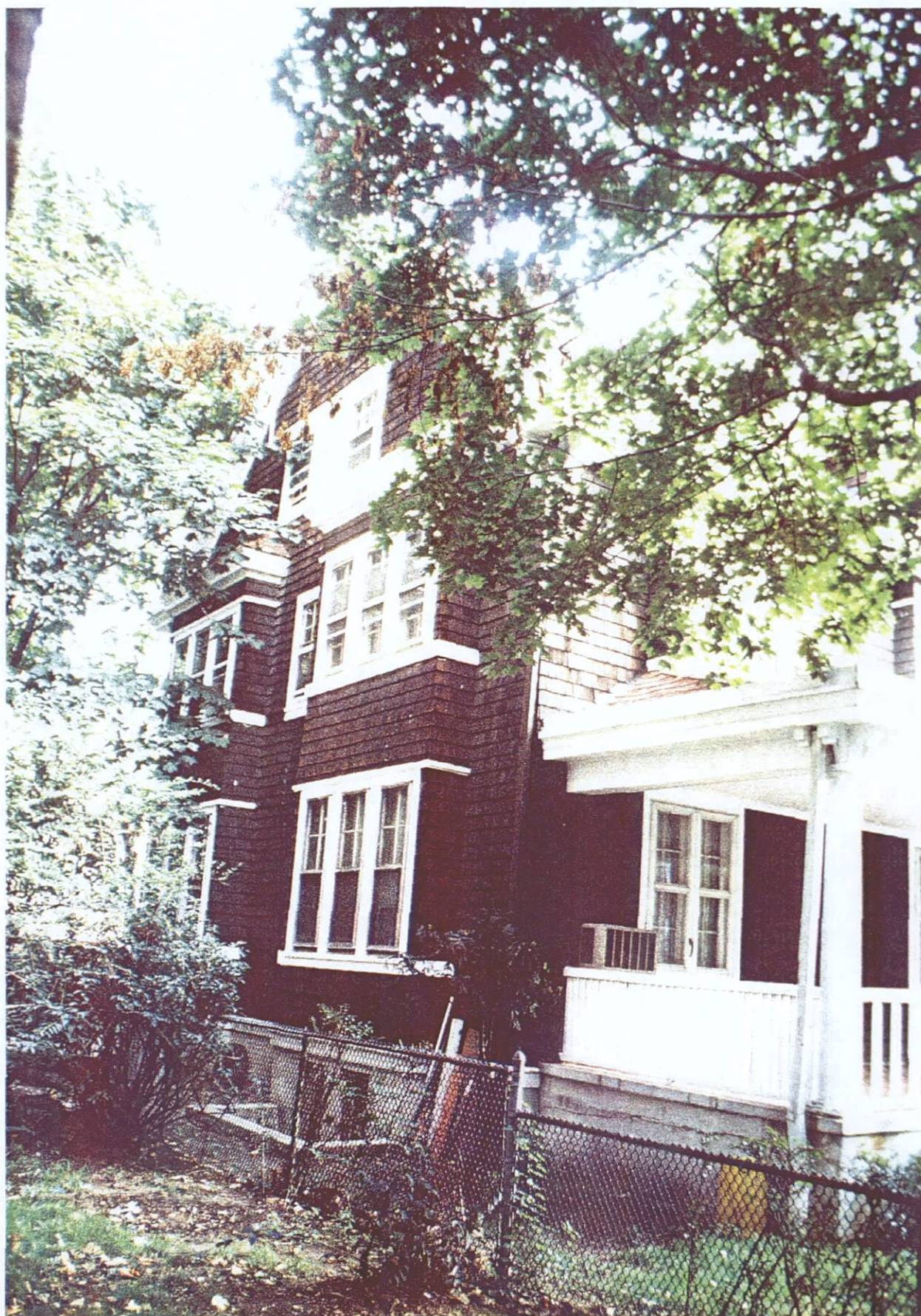
Figure 26. View of west side of Lot 86 2 1/2 story Church structure along fenceline, looking northeast from alley at rear of Vernon Apartments. Note recessed well with basement windows along west foundation wall.
