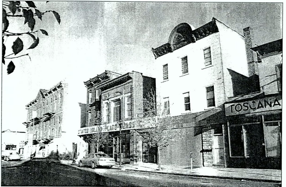
View northeast of commercial buildings located along Port Richmond Avenue
