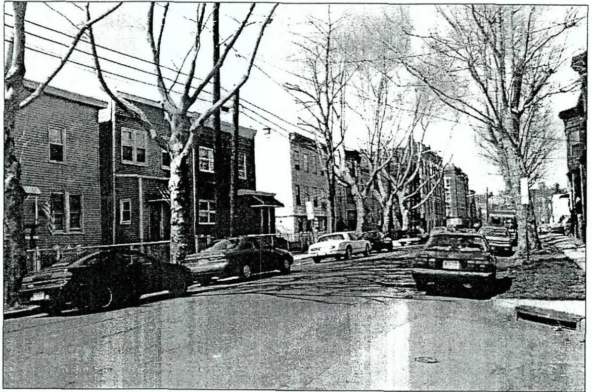
View northwest of residential development on Washburn Street
