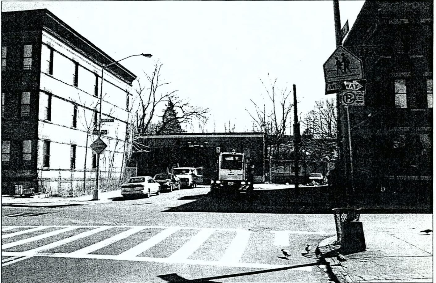
Wilson Avenue Station control house. View southeast on Wilson Street
