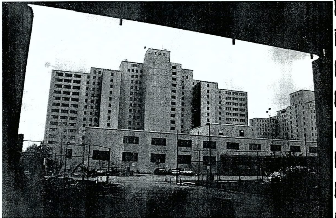
View west of Manhattan Psychiatric Center from beneath Triborough Bridge highway
