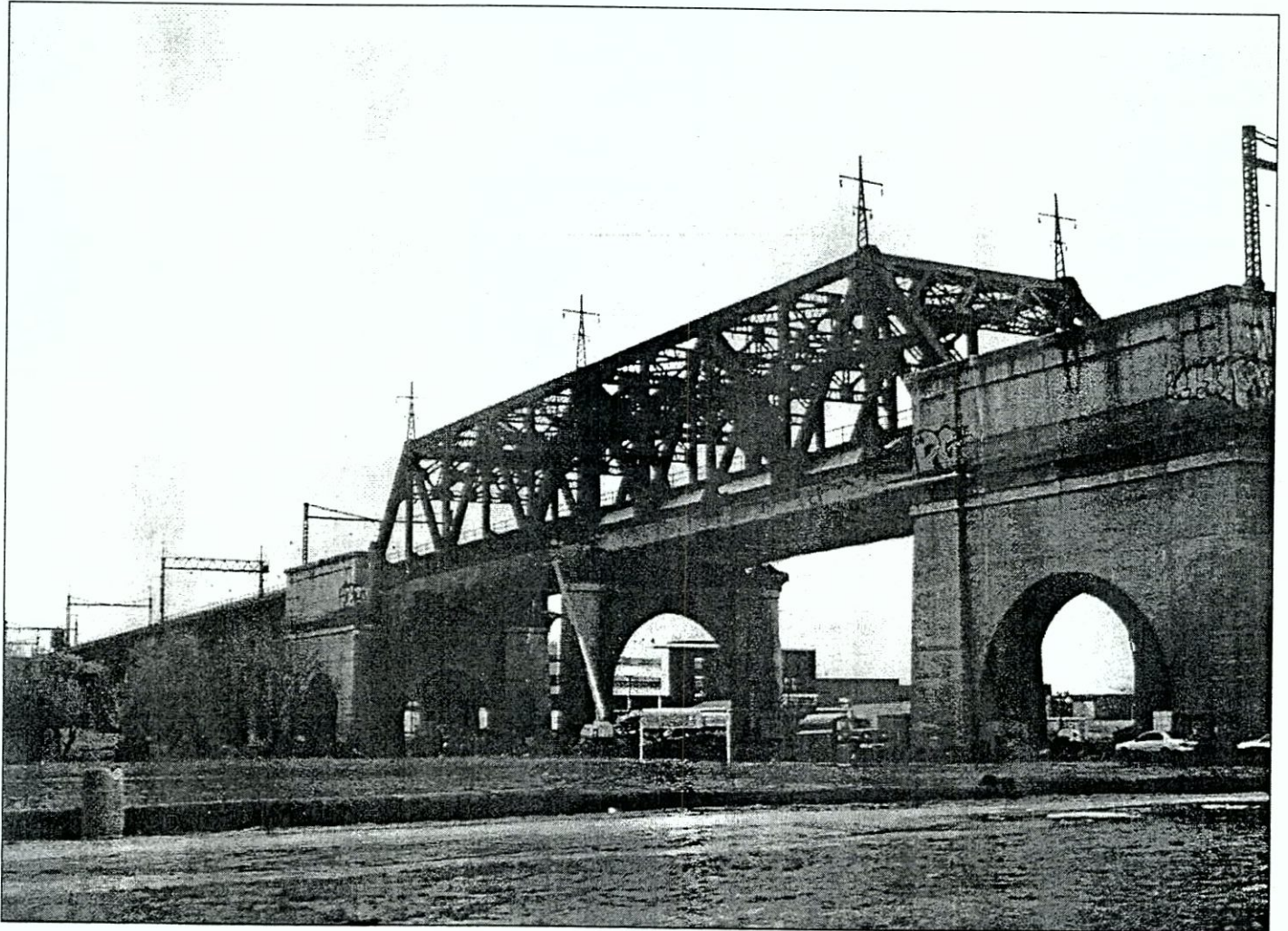
View east of Bronx Kill Bridge and Randalls Island playing fields
