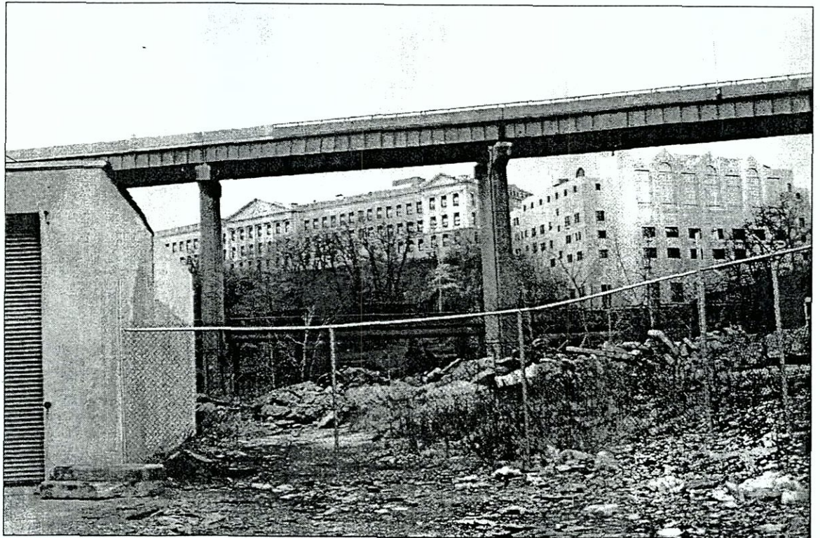
View northwest of an elevated portion of the rail line as seen from 10th Street. The New Jersey Turnpike Extension/I-78 travels overhead, while William Dickinson High School is visible in the background
