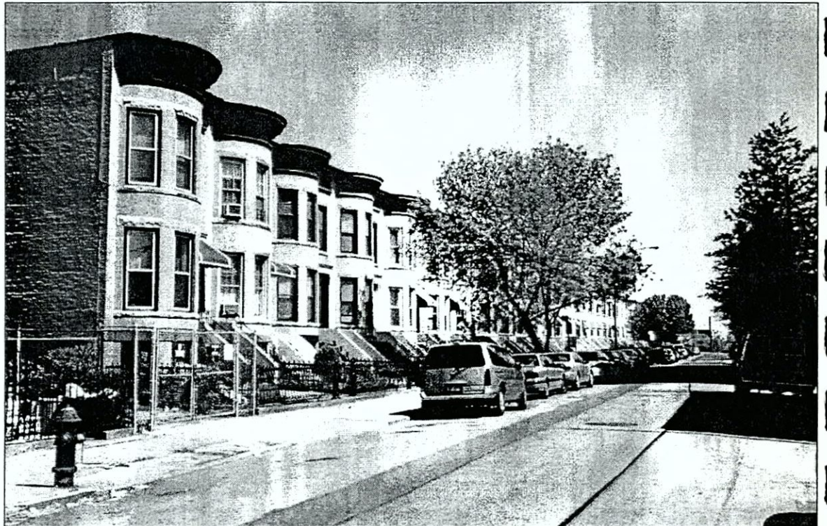
Sunset Park Historic District. North side of 64th Street between Fourth and Fifth Avenues. View east
