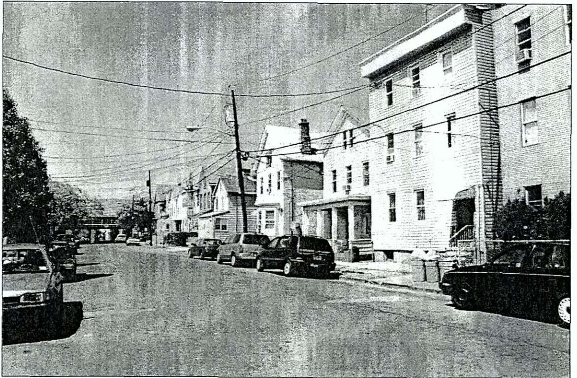
View north of Franklin Street, showing typical houses located in the study area. The elevated rail line is visible in the background
