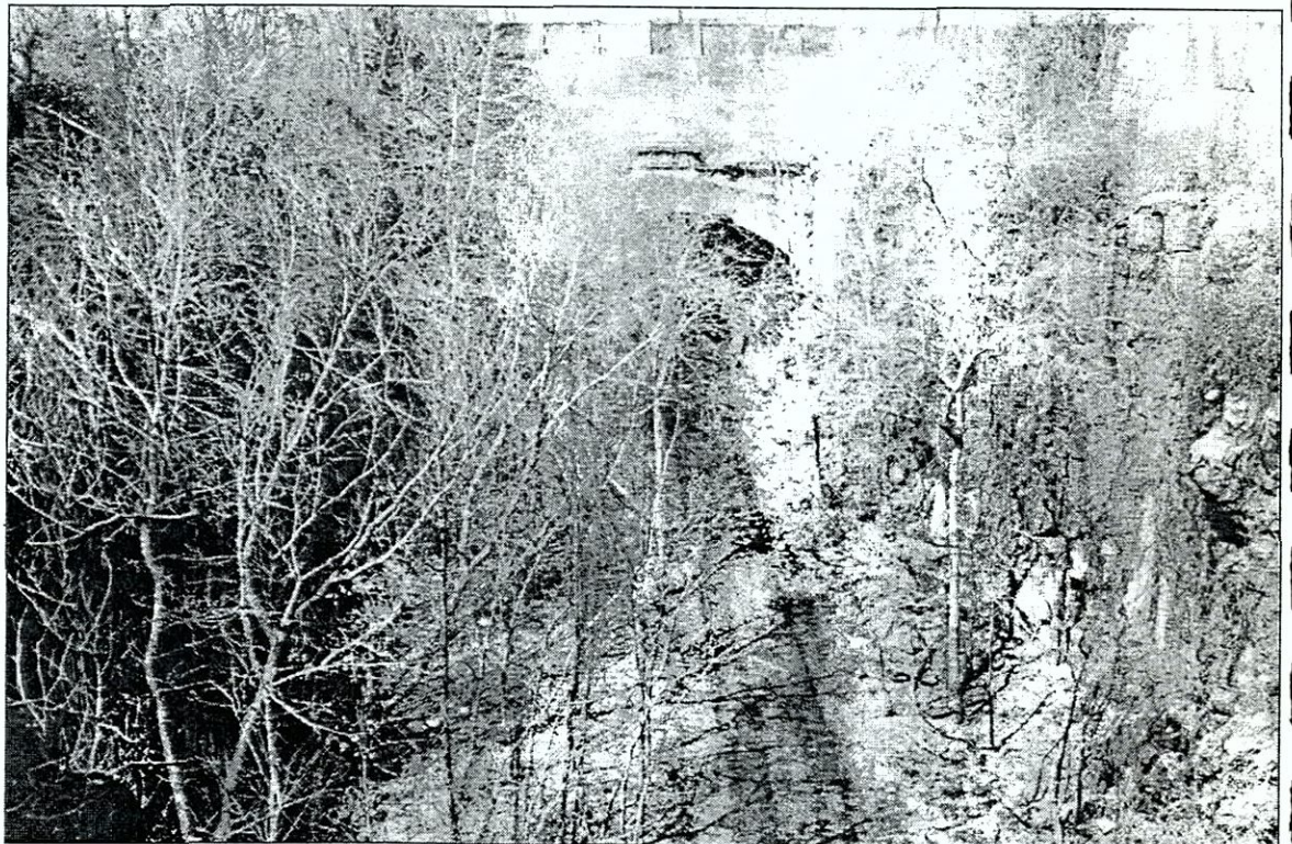
View northwest showing the Bergen Arches and Erie Cut as seen from Baldwin Avenue
