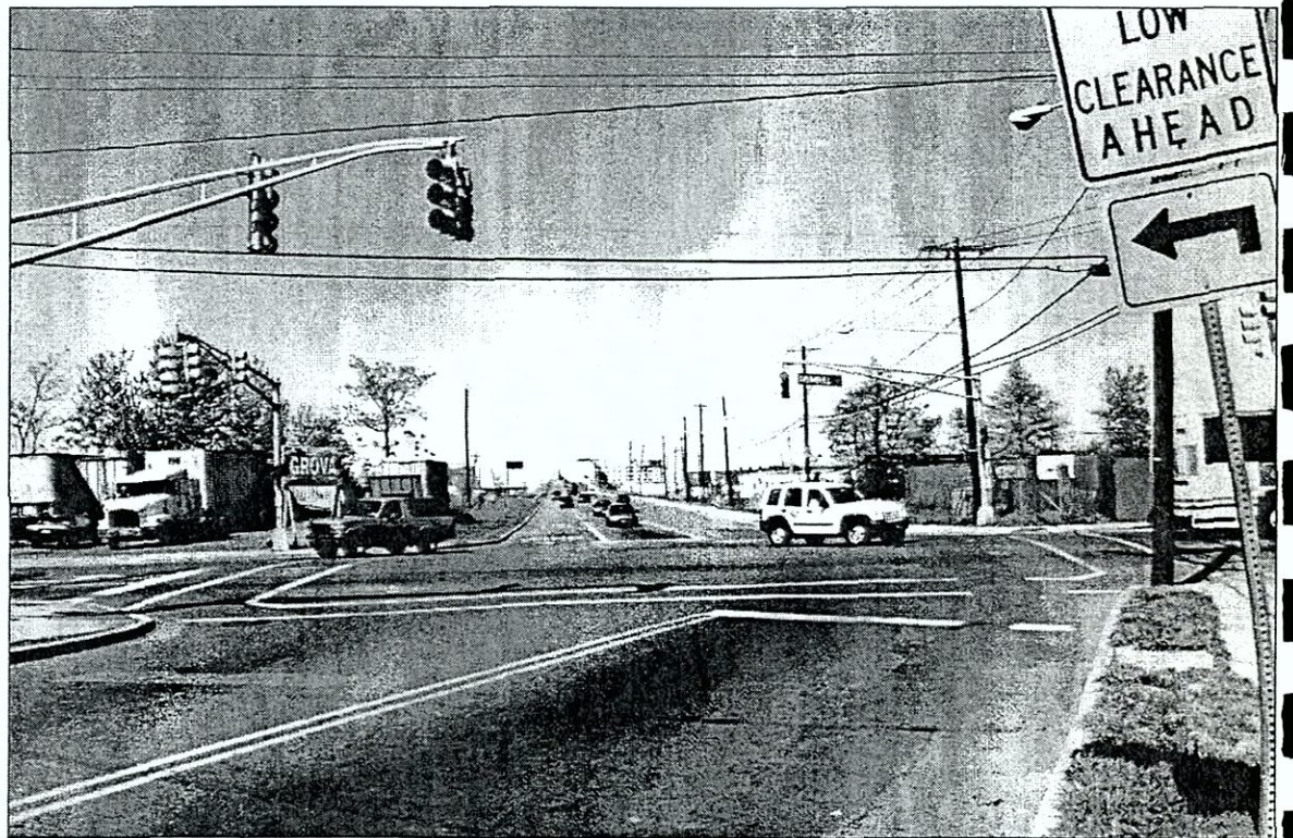
View northeast of the northern portion of the study area, as seen from the corner of Trumbull Street and 3rd Street
