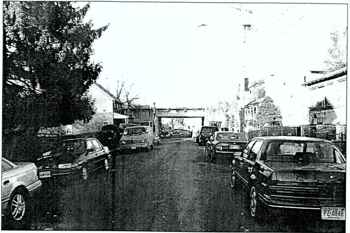
View north of the railroad trestle over Treadwell Avenue
