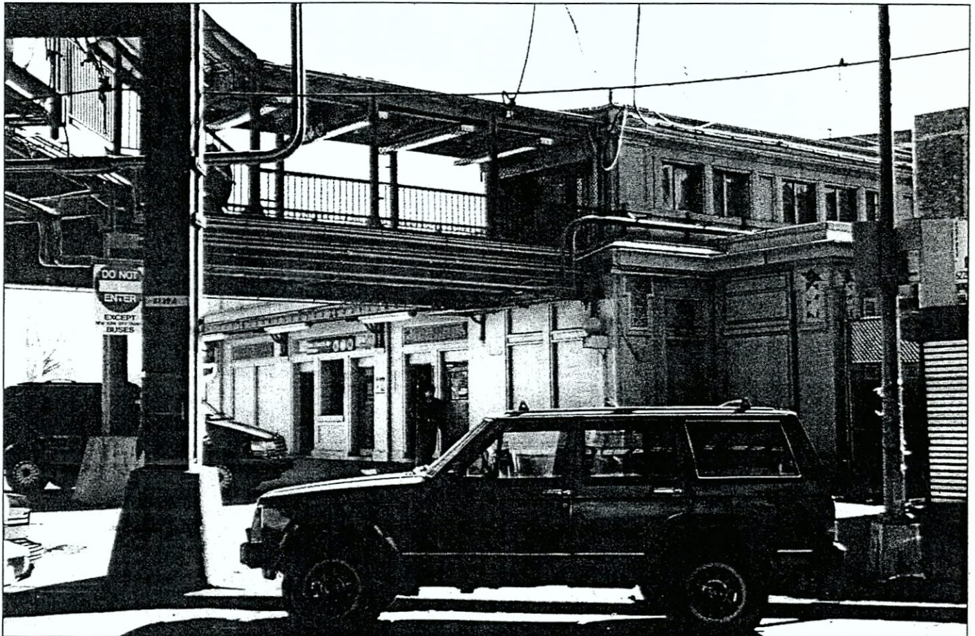
New Utrecht Avenue Station. View northeast
