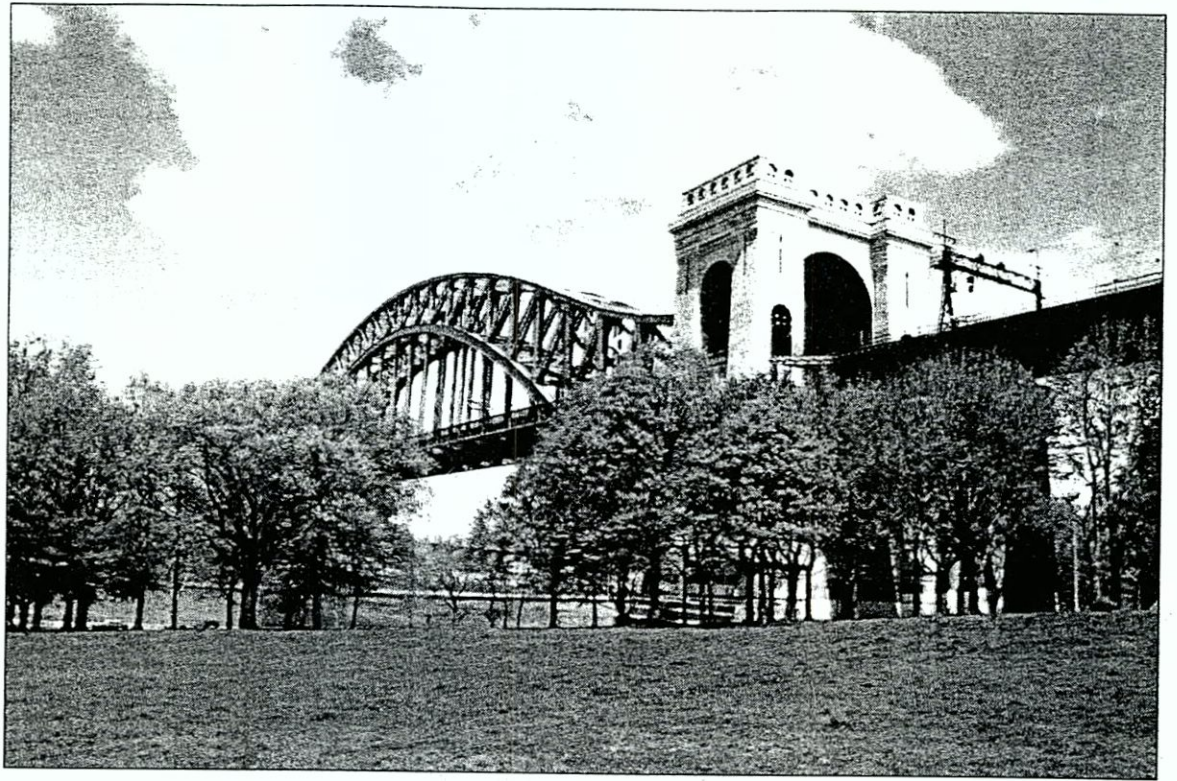
Hell Gate Bridge, view west from Astoria Park
