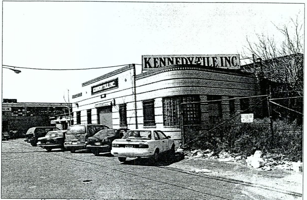
View southwest of the Kennedy Tile, Inc. building (a.k.a. the Roben Company Office Building), as seen from Tonnelle Avenue
