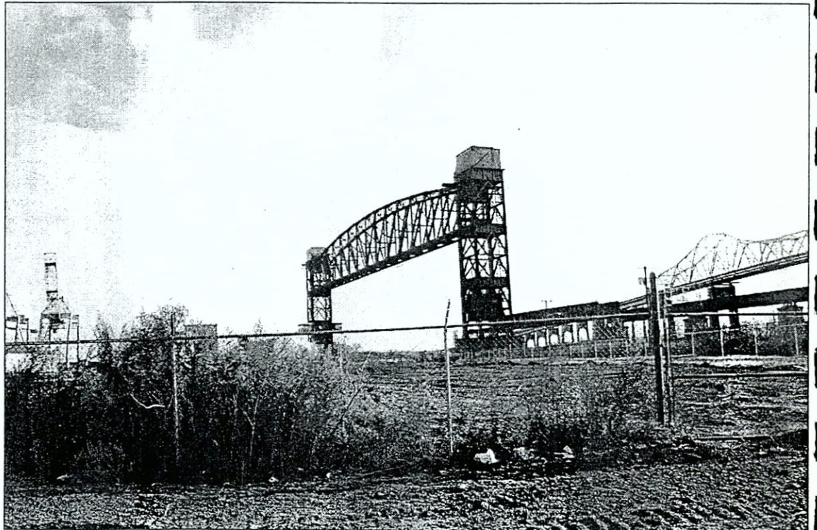
View south of the Arthur Kill Lift Bridge
