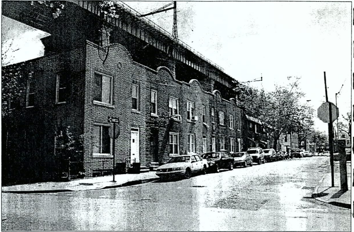
View east of 22nd Drive from 19th Street, with rail line above
