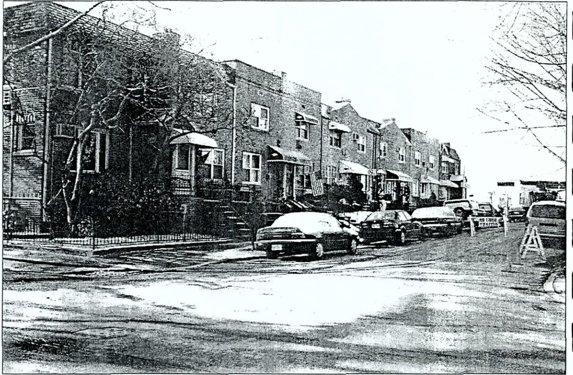
View west on Elmwood Avenue from East 3rd Street
