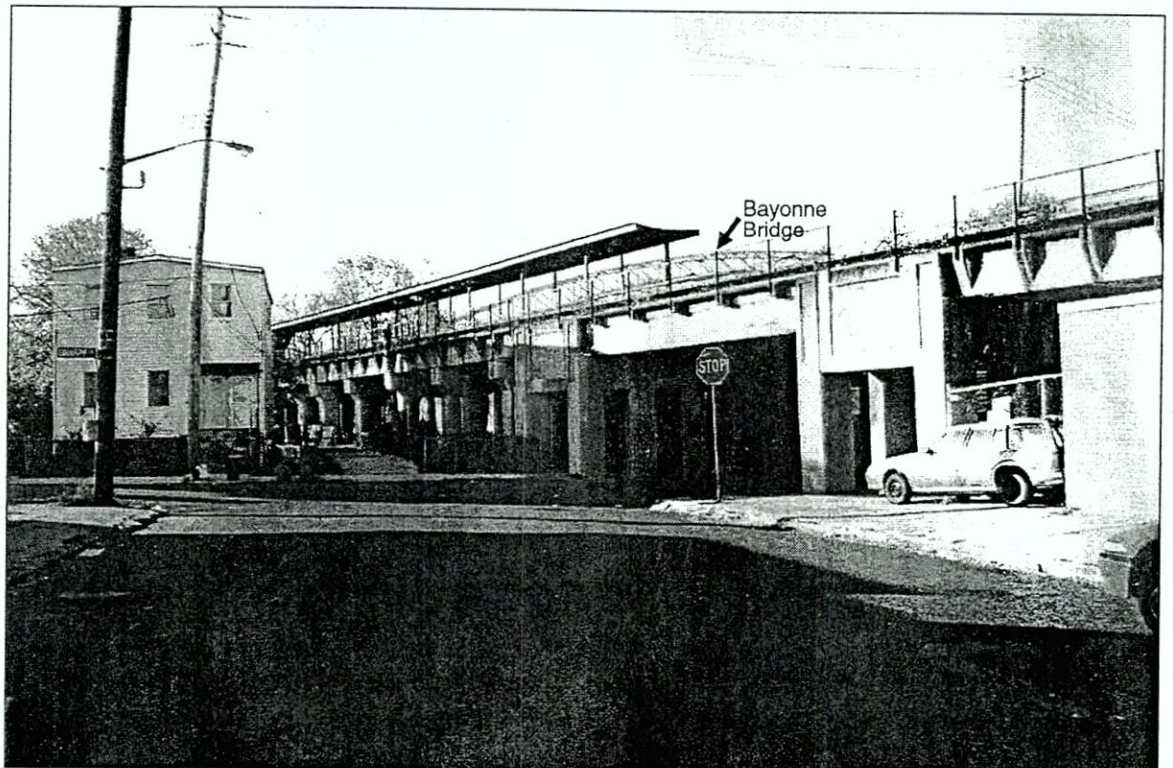
View northwest of the railroad trestle at Sharpe Avenue and Grove Avenue. The steel arch of the Bayonne Bridge is visible in the background
