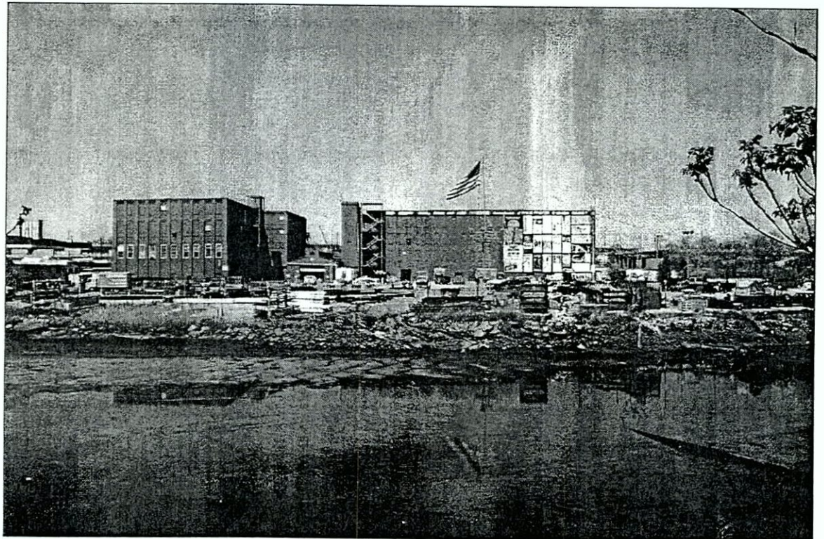
View north toward project site from south side of Maspeth Creek
