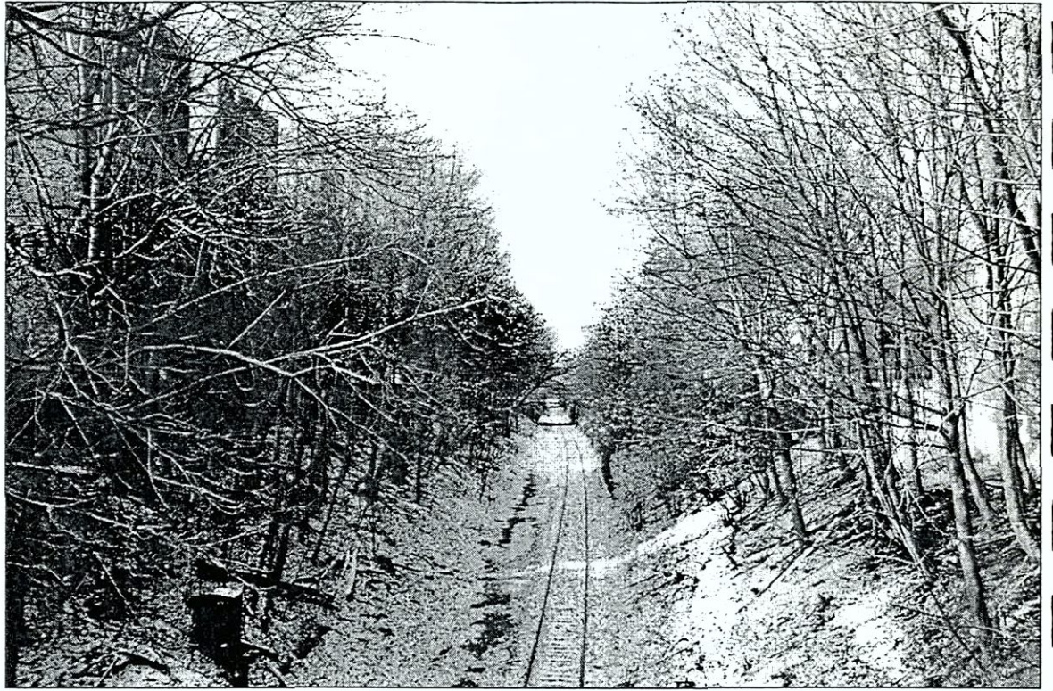
Bay Ridge Branch rail cut. View west from Ocean Parkway
