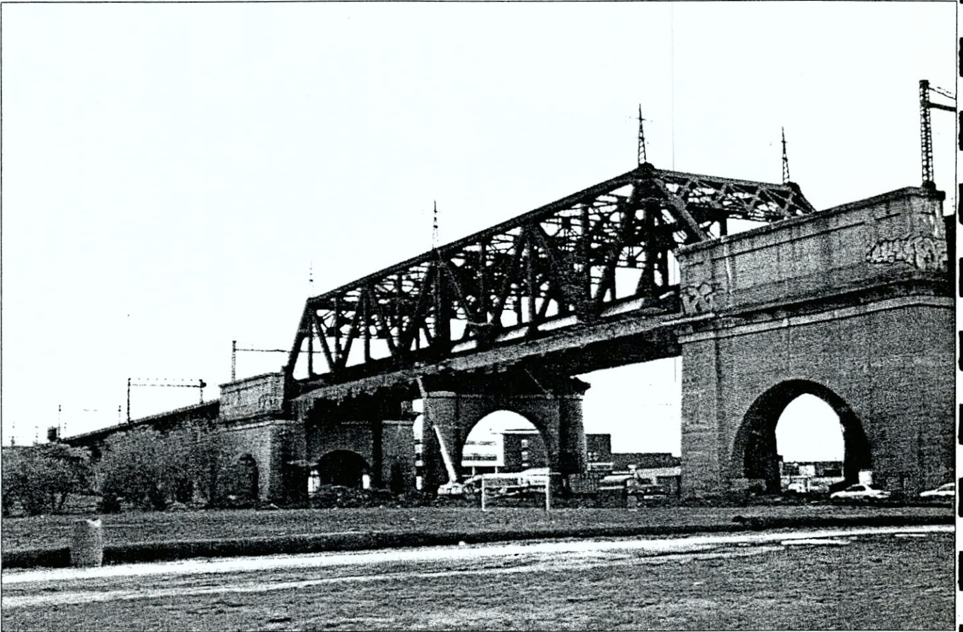
Bronx Kill Bridge, view east from Randalls Island
