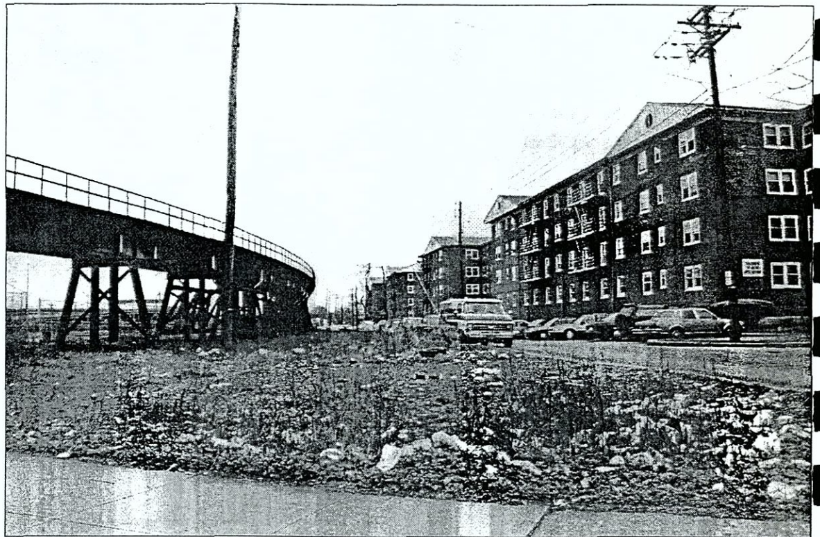
View southeast of the rail line as it is carried by a trestle, near Merseles Street
