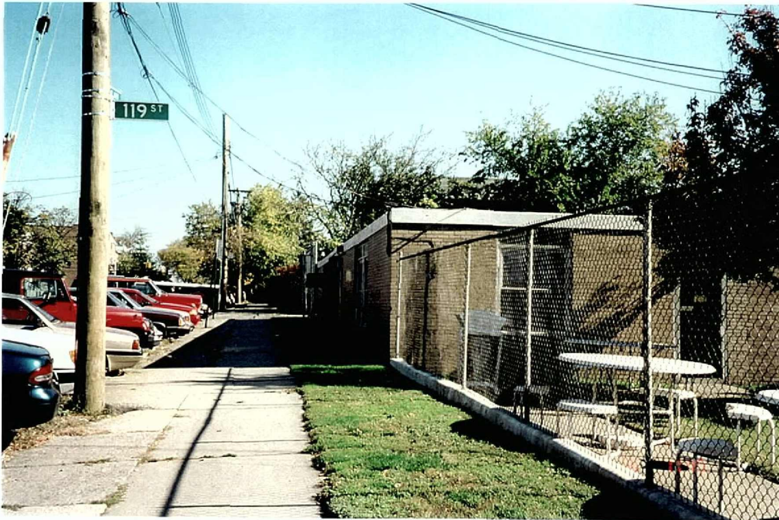
Photograph C. North side of Nursing Care Center. Building in background is to be razed, proposed new building to be set back 20' and cover patio (facing east along 26 th Avenue).
