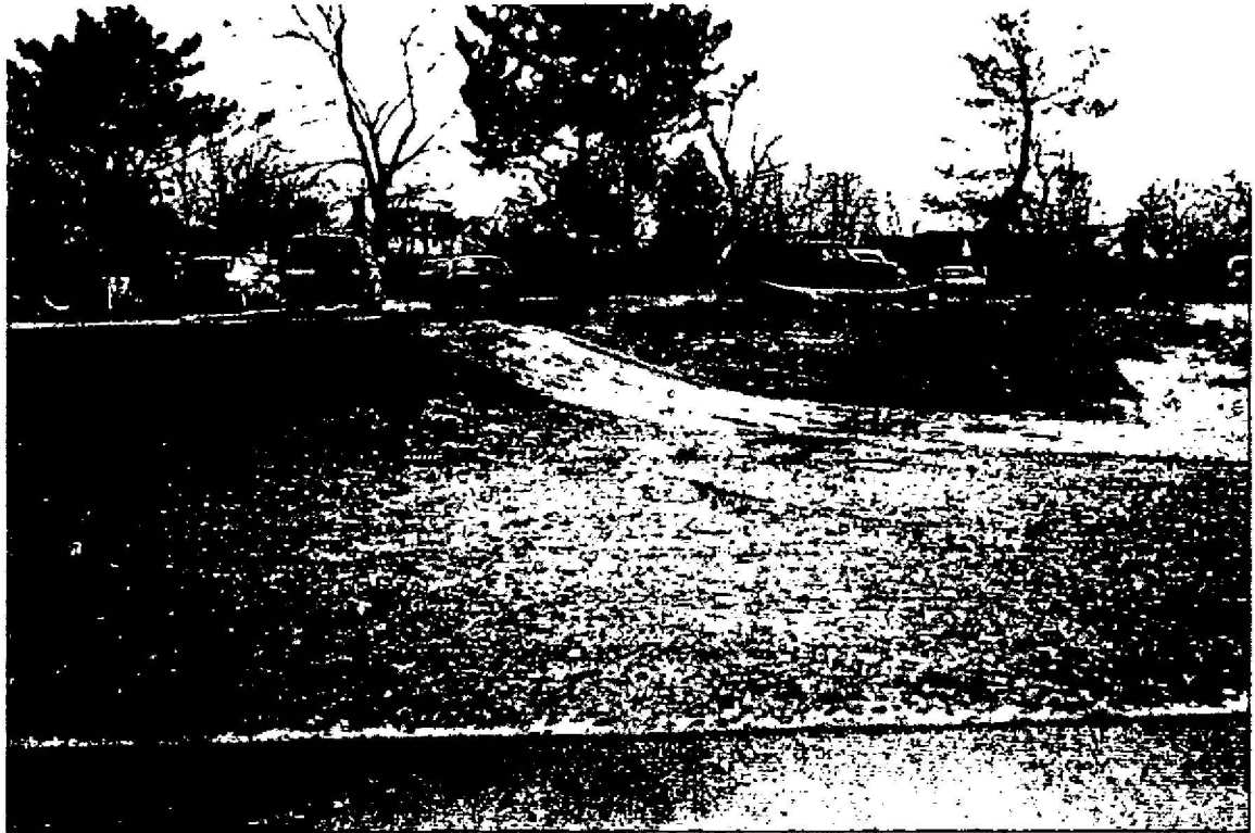
Photograph A St. John's University Parking Expansion Project Site View: north to south
